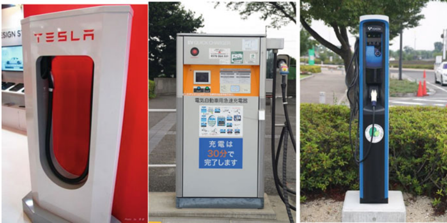
Fig. 8 Examples of charging equipment for BEVs/PHEVs (left: TESLA supercharger, middle: quick charger, Right: 200-V normal charger)
