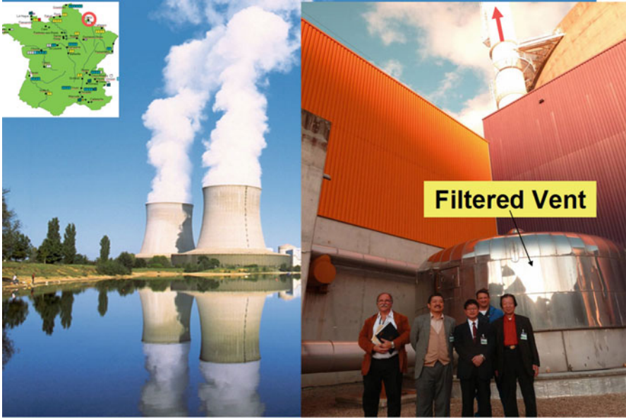
Fig. 19 FCVS installed in Chooz NPP (PWR), France [8]
