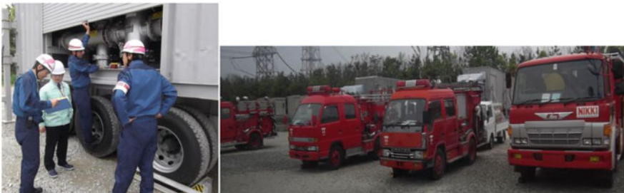
Fig. 34 Examples of tsunami protection measures at NPSs [14]. (a) Gas turbine generator at Shimane NPS. (b) Oil tank at Shimane NPS. (c) Snorkel building at Shimane NPS (d) Large wall, door and balconies at Kashiwazaki-Kariwa NPS. (e) Mobile cooling car and fire engines at Kashiwazaki-Kariwa NPS
