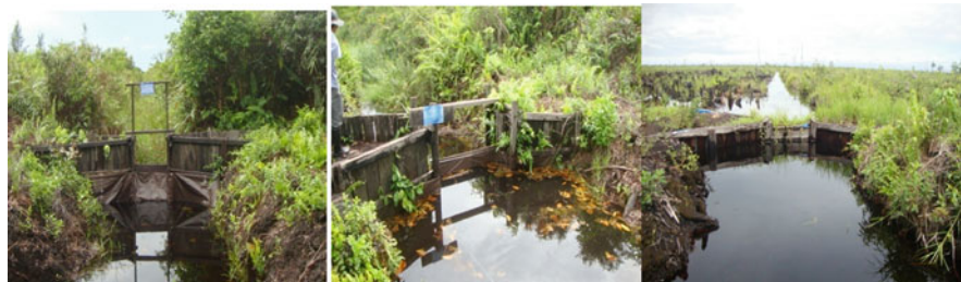
Fig. 34.2 Floodgates or tabat are very important in maintaining water levels of peatlands (Noor 2011)
