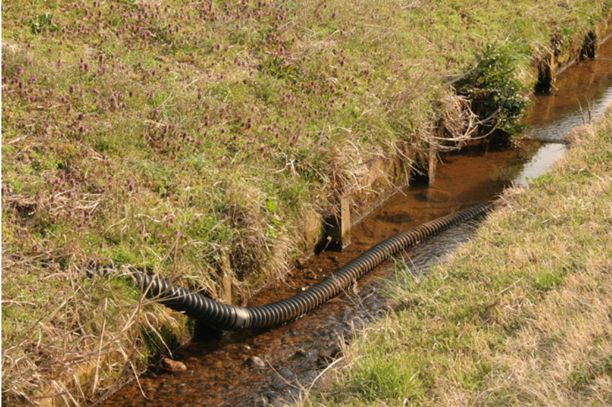
Fig. 5.7 A fishway constructed from a corrugated pipe to increase habitat connectivity between a paddy field and its adjacent drainage
