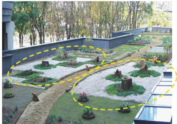
Fig. 10.15 Oita city hall rooftop greening
