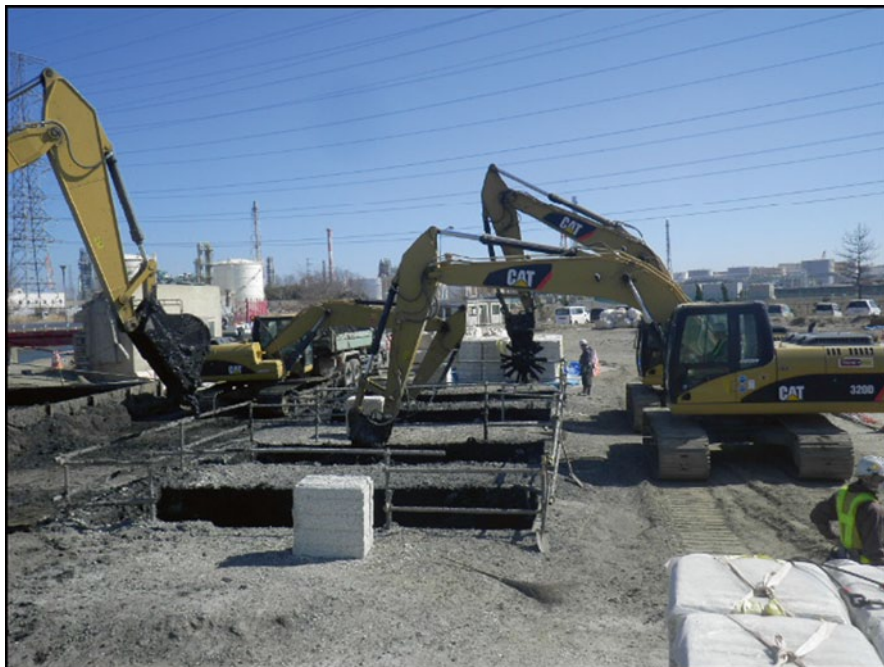
Fig. 10.11 Condition improvement using fiber-cement stabilized soil-based construction at Sunaoshi river, Tamajo, Miyagi Prefecture
