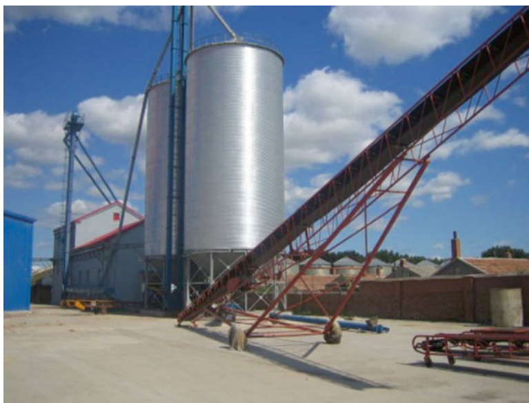
Fig. 13.7 Temporary storage facility for unprocessed rice
