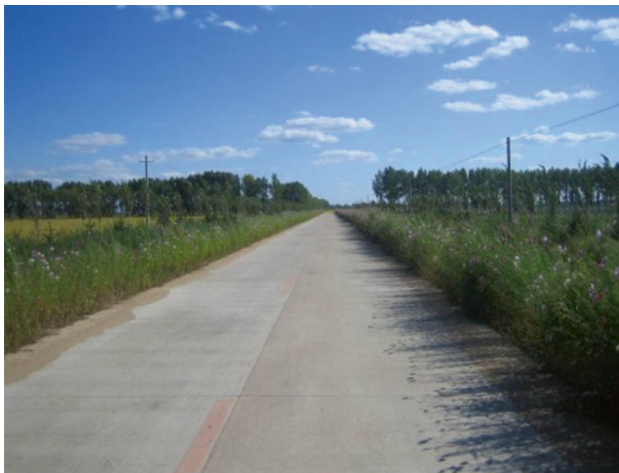
Fig. 13.2 Paved farm road
