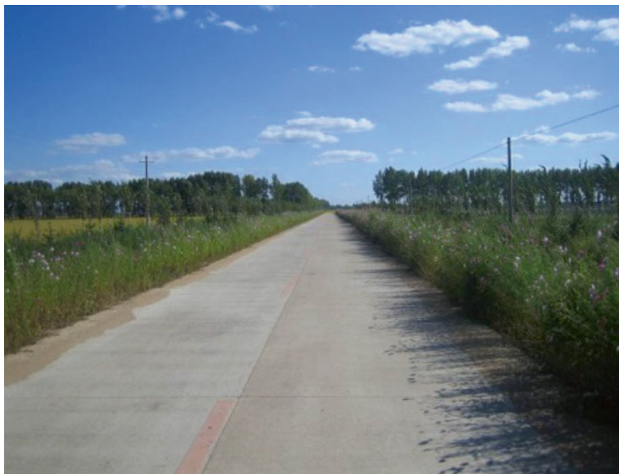
Fig. 13.2 Paved farm road
