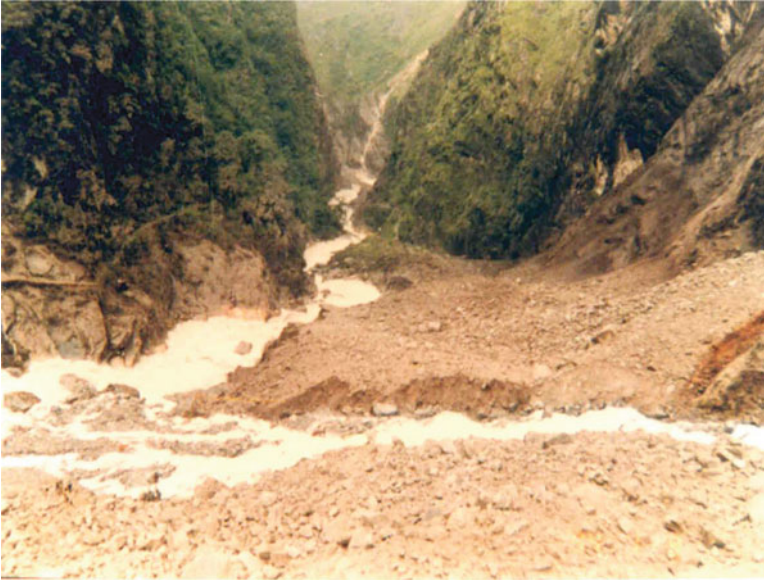
Fig. 12.5 Post-disaster view of Malpa Landslide site
