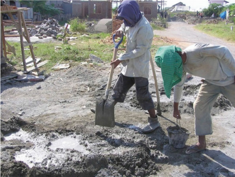
Fig. 17.2 Local builders in housing reconstruction
