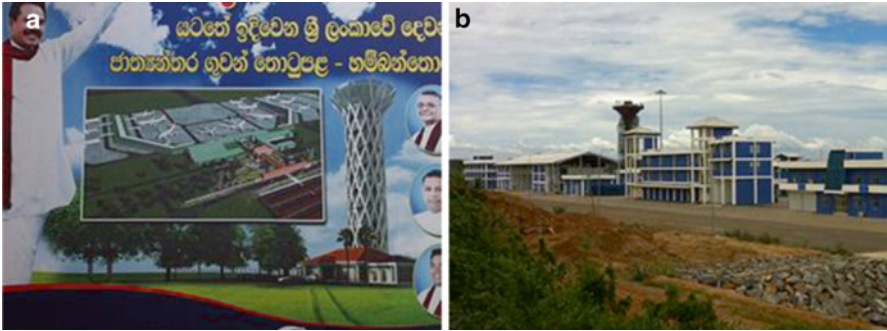
Fig. 6.9 Large projects in Hambantota, Sri Lanka. (a) International airport. (b) International ferry terminal
