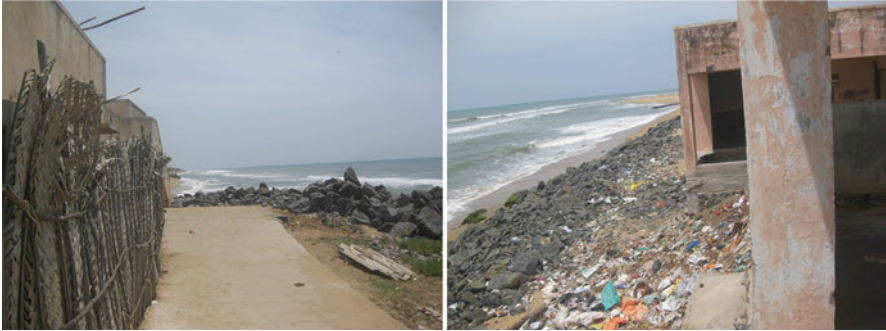
Fig. 24.12 Few pockets of coastal villages are undergoing shore erosion recently
