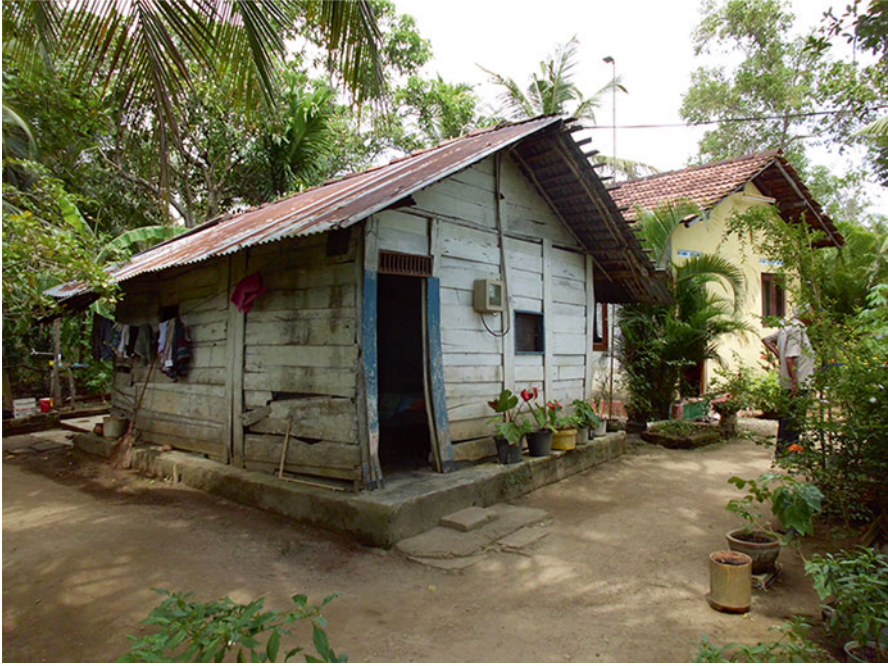
Fig. 27.4 Flimsy houses such as this was typical in the area before the tsunami. Note in the background the much better type of house built by HfH-SL
