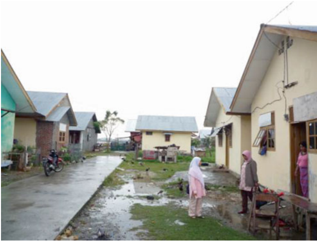
Fig. 15.3 Newly constructed houses in one community
