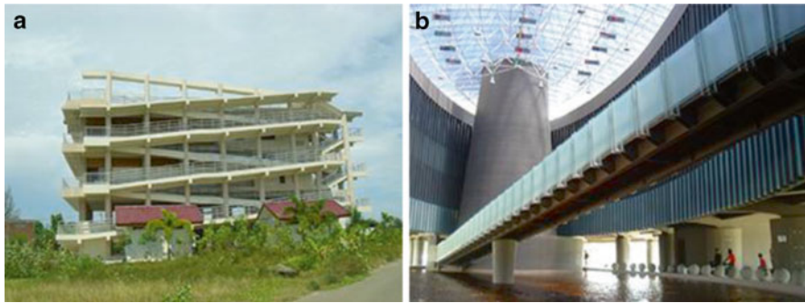
Fig. 6.11 New facilities in Banda Aceh, Indonesia. (a) Community building. (b) Aceh Tsunami Museum
