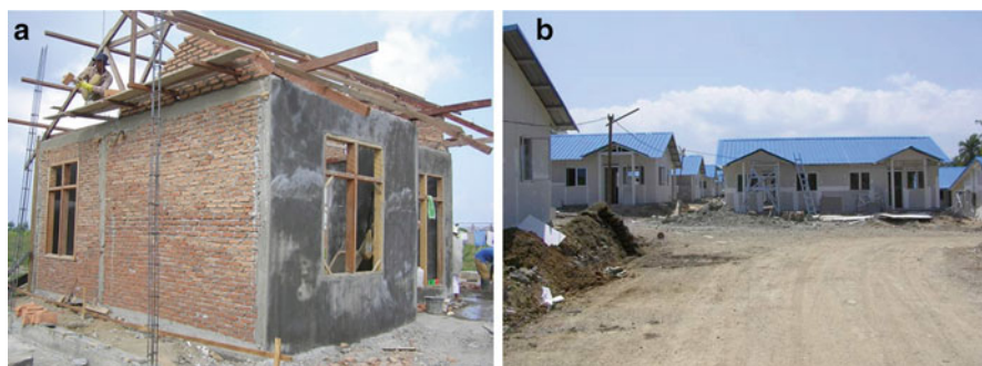
Fig. 17.1 (a) Type 36 houses under construction by BRR. (b) Houses with imported materials
