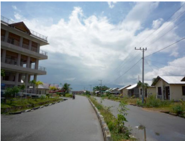
Fig. 15.4 Tsunami evacuation tower and widened-paved road
