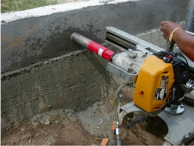
Fig. 16.9 Concrete core sample for test
