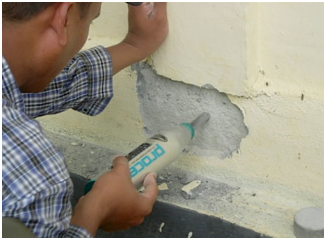
Fig. 16.7 Schmidt hammer Test
