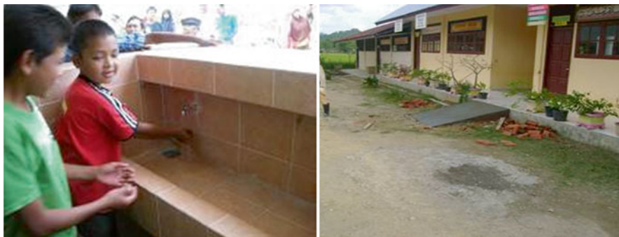
Fig. 16.13 Child friendly features—Hand wash sink and ramp for disable
