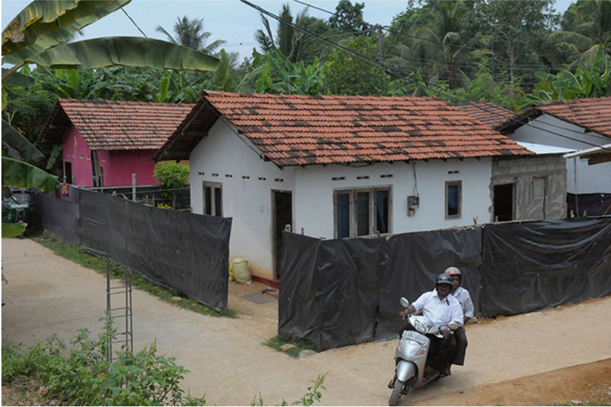
Fig. 27.3 Houses built by HfH-SL in Galle
