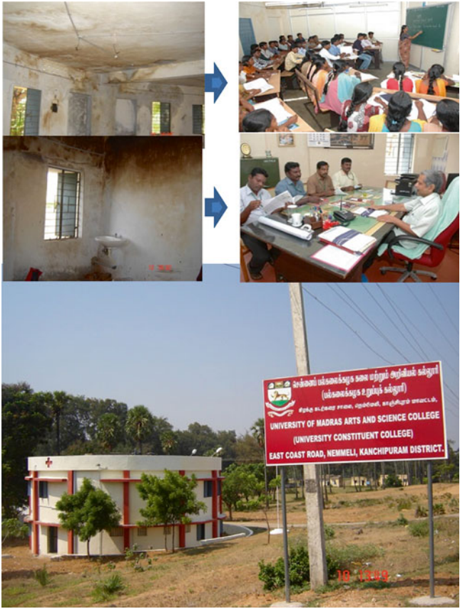
Fig. 24.1 Converted cyclone shelter for the college
