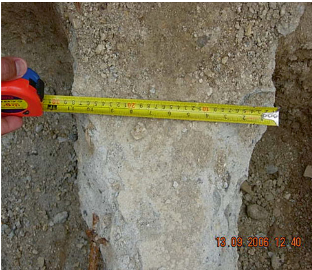
Fig. 16.4 Size of member less than required
