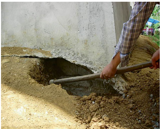
Fig. 16.6 Verification of foundation
