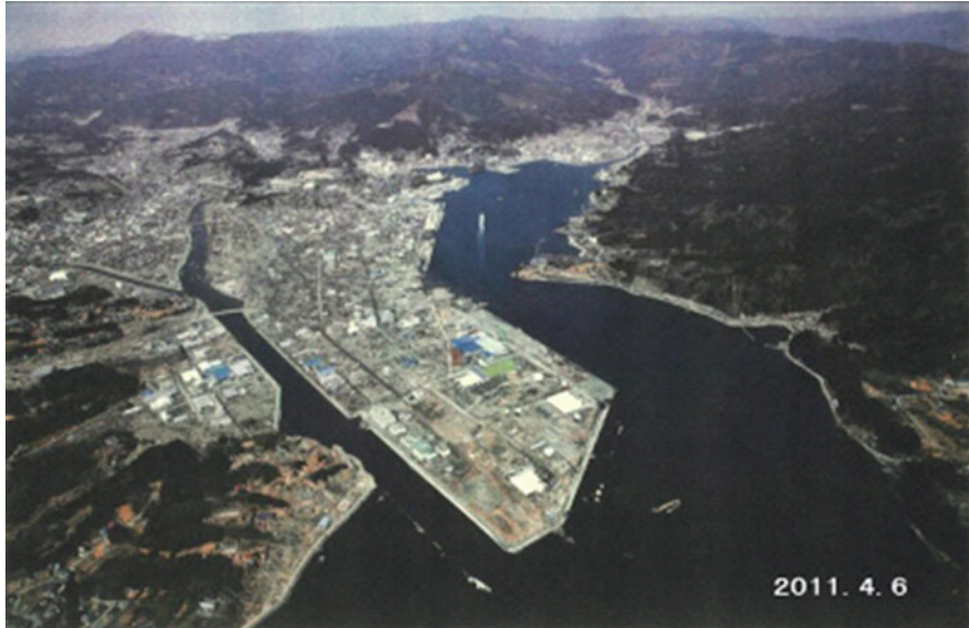
Fig. 7.5 Damage by disaster (Tsunami) in Minami Kesennuma district in Kesennuma ( Source: A. Sugawara )
