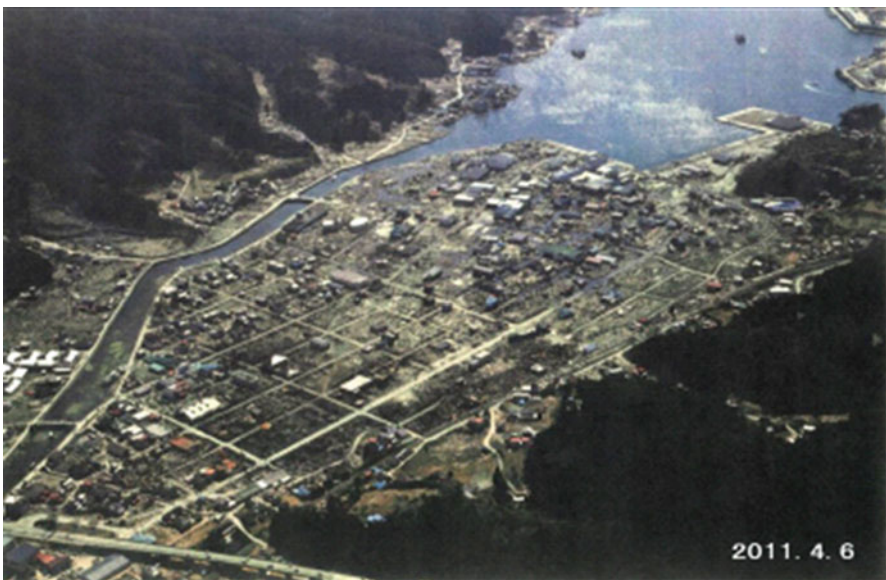
Fig. 7.4 Damage by disaster (Tsunami and fire) in ShiShiori district in Kesenuma (Source: A. Sugawara)
