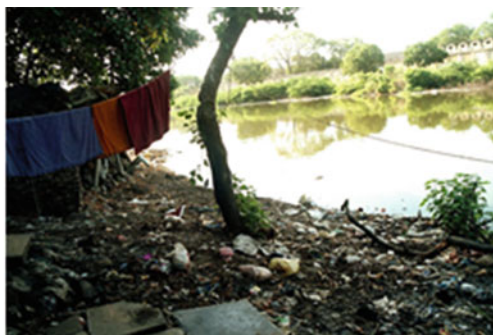
Anjukudisai Slum, Chennai: a narrow street in 2004 – note drainage and restricted space for people's use
