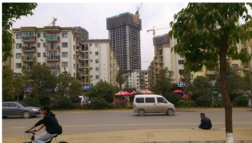
Fig. 17.15 An example of low rental housing—XingFuYuan (Happy Family) (photo taken by Guihua Chen in 2013)
