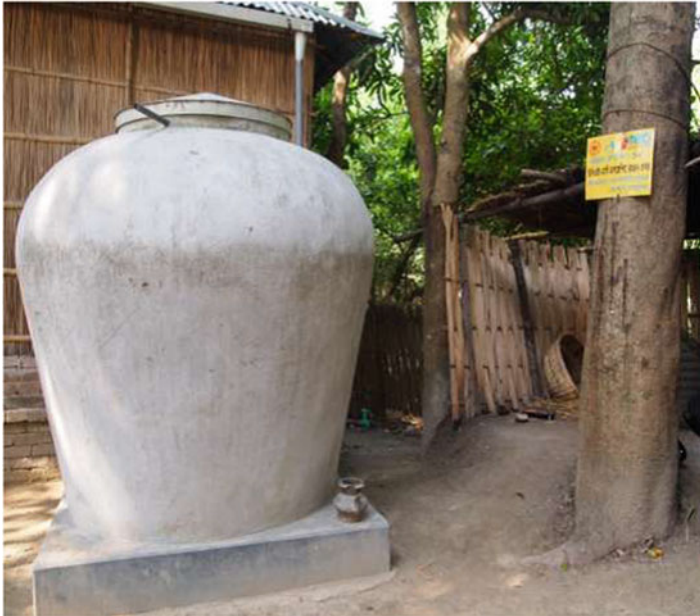
Fig. 9.3 Rainwater harvesting unit
