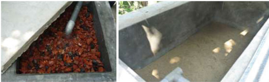
Fig. 9.4 River sand filter unit
