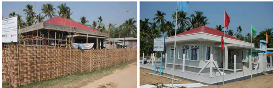
Fig. 13.4 Health center with cyclone-proof structure by MERCY Malaysia
