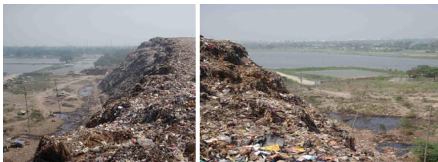
Fig. 21.3 Leachate ponding at Dhapa disposal site
