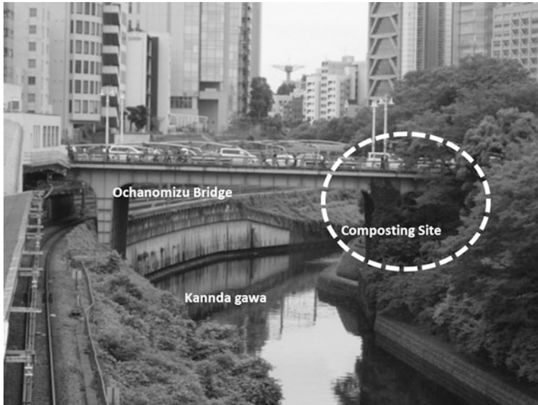
Fig. 3.8 Composting site under the Ochanomizu Bridge. (Photograph by Kato 2011.6.15)
