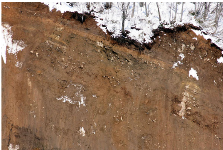
Fig. 11.7 Tuff and andesite with developed cracks exposed at the head scarp
