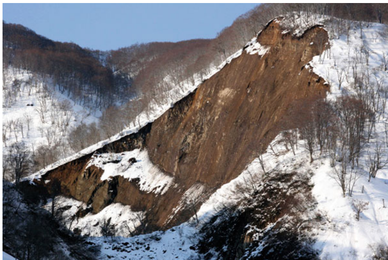
Fig. 11.6 Deep-seated landslide on the left bank of the Higashi-irisawagawa River
