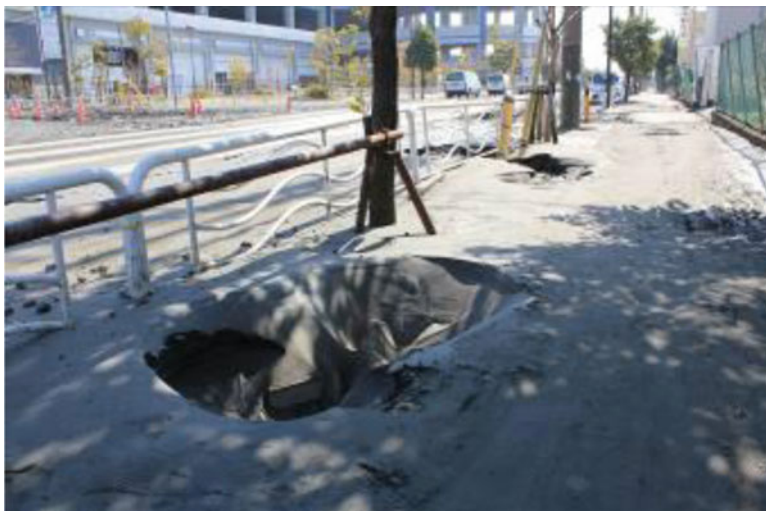
Fig. 10.23 Sand accumulated on a sidewalk
