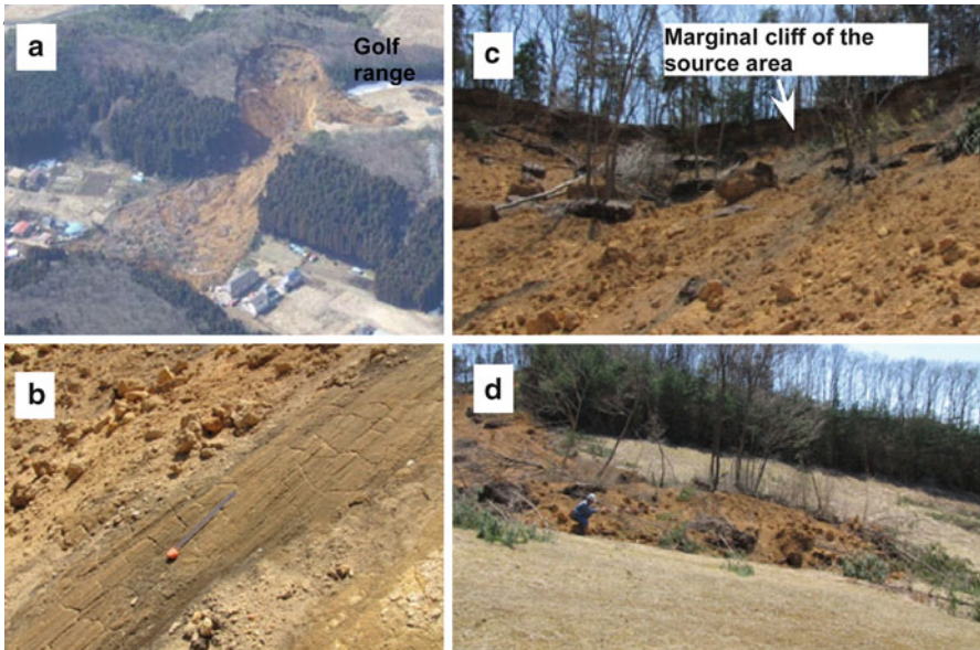
Fig. 6.3 Photographs of the Hanokidaira landslide. (a) Overview (photo by the Ministry of Land, Infrastructure, Transportation and Tourism); (b) sliding surface (c) standing trees remaining in the source area; (d) landslide deposits on the turf in a golf range
