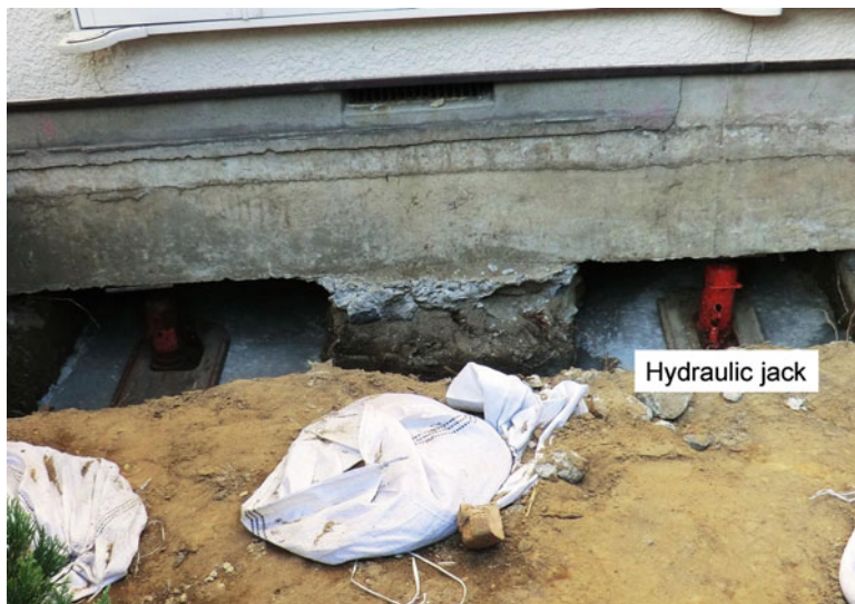
Fig. 10.22 Example of jack-up technique
