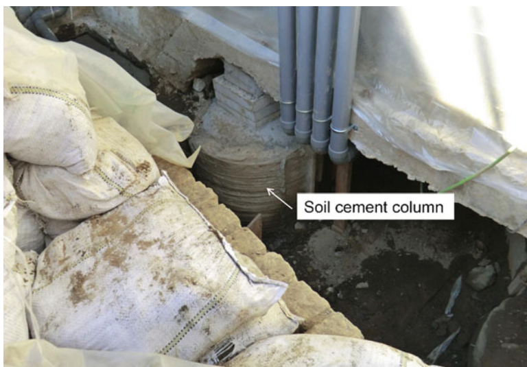
Fig. 10.18 Soil cement column
