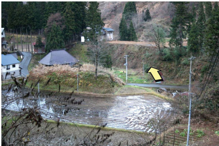
Fig. 11.12 Akakura landslide after earth removal works (view from the south)
