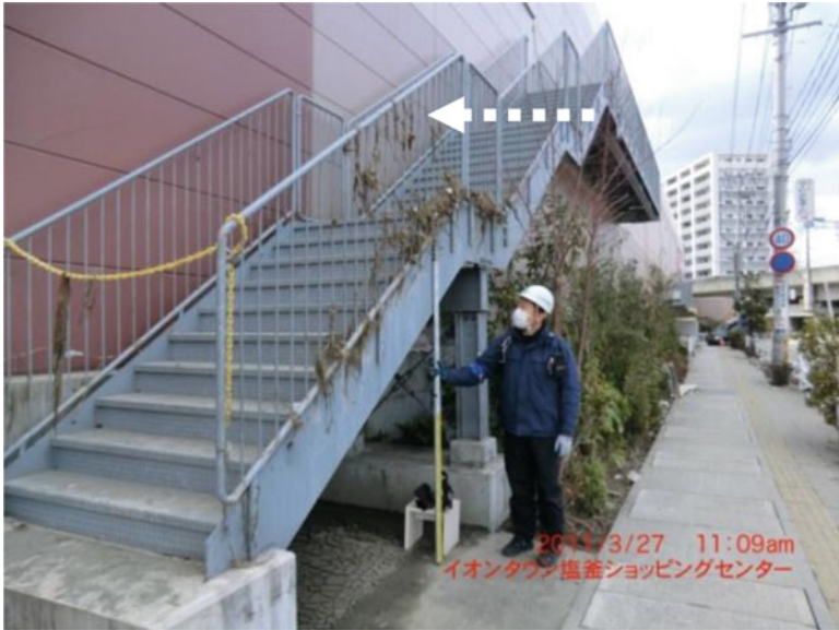
Fig. 4.10 Evidence of tsunami height left at a shopping center
