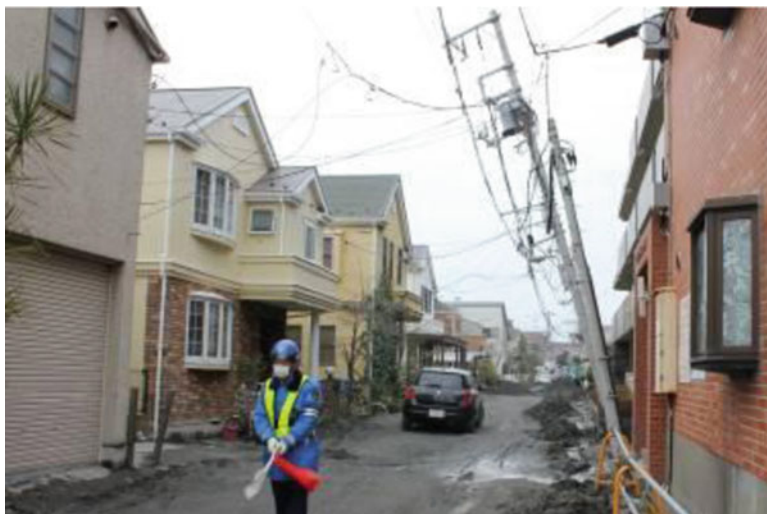
Fig. 10.4 Residential area covered by sand from a sand boil
