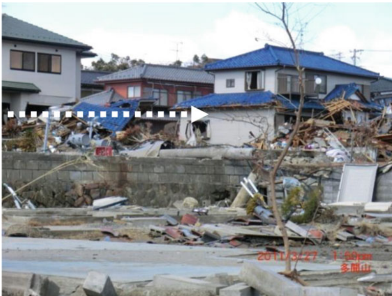
Fig. 4.11 Damaged wooden houses on the Shobutahama coast
