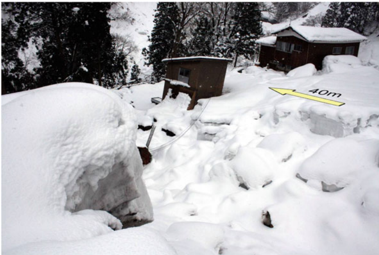
Fig. 11.9 Reactivated landslide moved approximately 40 m during the earthquake
