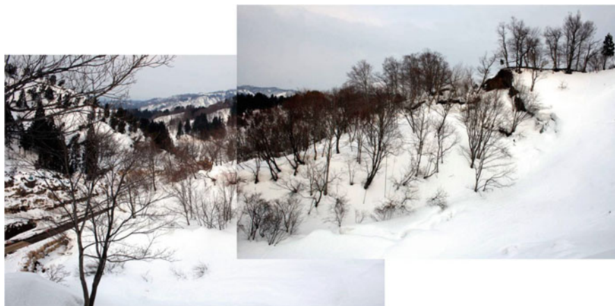
Fig. 11.14 Side view of the landslide in Tsukiike
