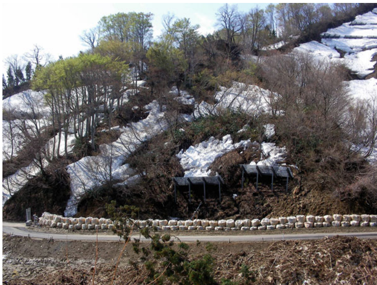
Fig. 11.15 Front view of the landslide in Tsukiike
