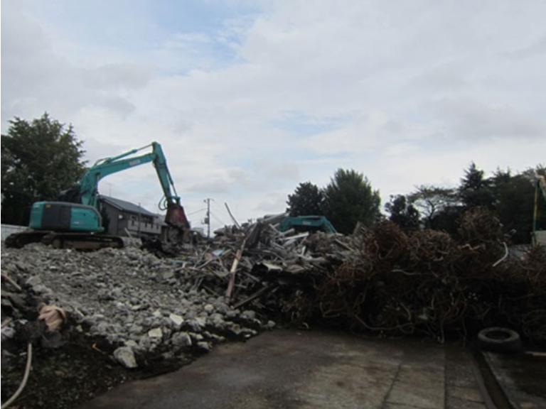
Fig. 3.17 The demolish of government officers' apartment in December 2012
