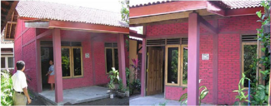
Fig. 11.4 A reconstructed house was built according to earthquake resistant house manual by a local university in Yogyakarta ( Source : Pribadi et al. 2008)
