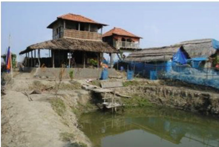
Fig. 13.9 A house modified by the owner (photo: Hasibul Kabir)
