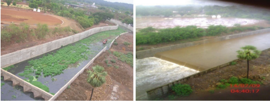
Fig. 15.8 Detention pond allows low flows to flow through but stores high rainfall intensity flows and allows overflows
