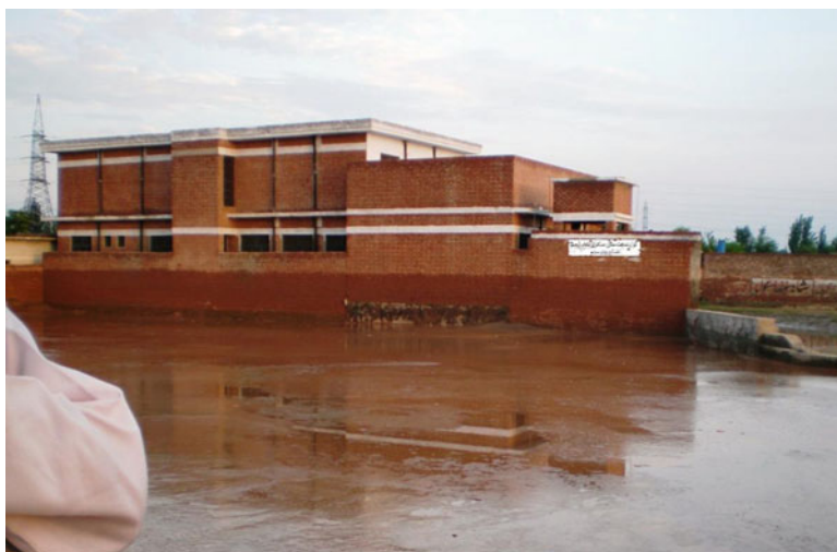
Fig. 7.3 Middle school affected by floods: 2010
