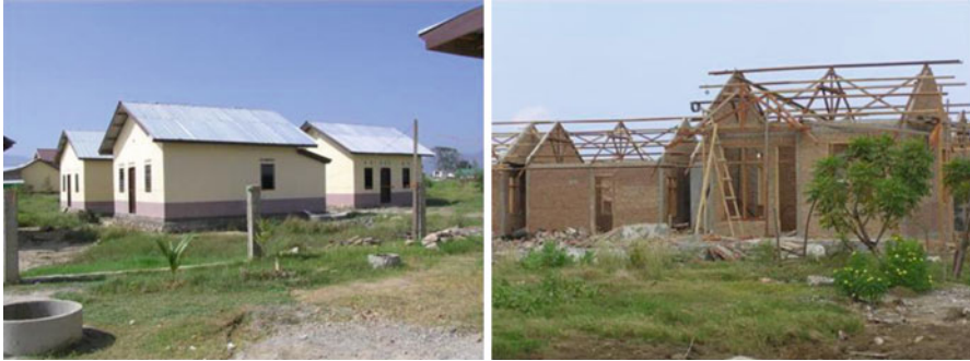
Fig. 11.2 A post-tsunami housing reconstruction project ( source : Field Observation in Banda Aceh 2006)
