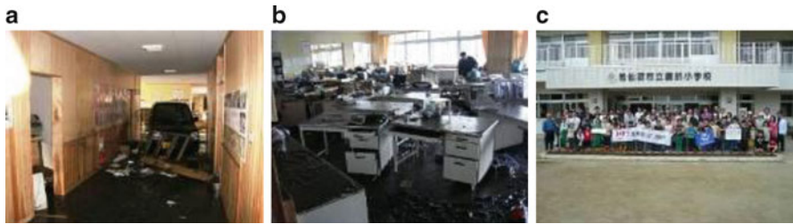
Fig. 6.4 (a) Hallway in front of principal room, (b) Staff Room destroyed by tsunami, (c) School Garden Recovery Project with volunteers of bank
