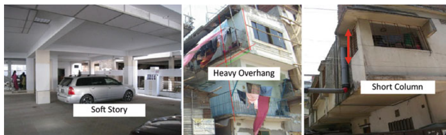
Fig. 6.8 Vulnerability factors of buildings frequently observed in Bangladesh
