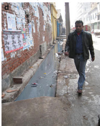
d Chemical and waste from tannery industry are passing through open drain, which over flow during rainy season (Zone No. 3)
