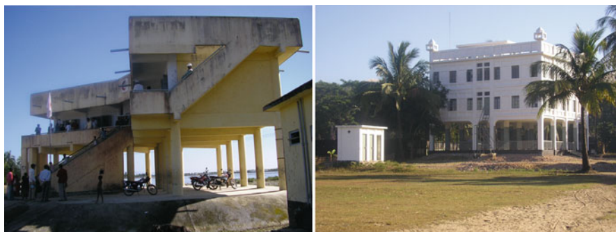
Fig. 5.2 Traditional cyclone shelters in Bangladesh ( Source: Postgraduate Programs in Disaster Management, BRAC University)
