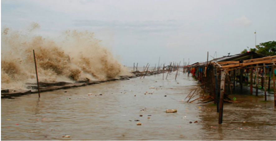
Fig. 8.4 Storm surge destroying coastal area of Patengasea beach
