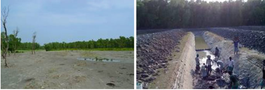
Fig. 15.1 Periodically inundated and fallow coastal lands are arranged for ditch and dyke uses
