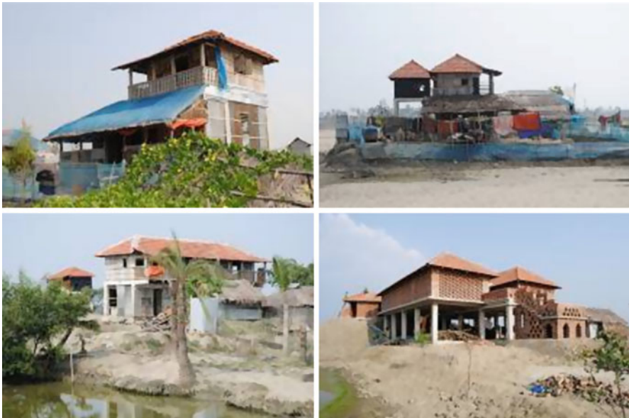
Fig. 17.7 Independent modifications and extensions at the post-basic construction phase. The bottom-right is the photograph of the school-cum common shelter. Source: Khandoker Hasibul Kabir, Department of Architecture, BRAC University
