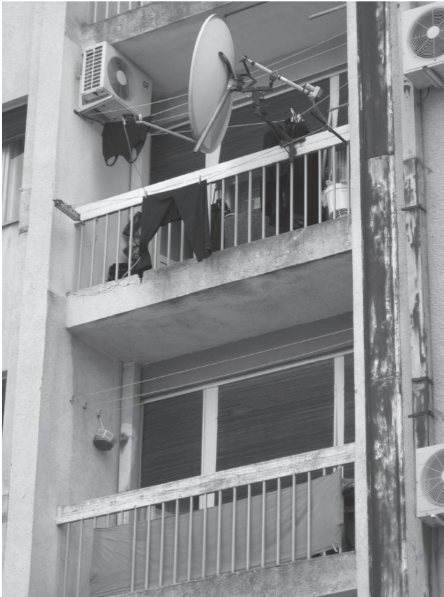
Fig. 7.3 Low income multi-apartment homes in Skopje
