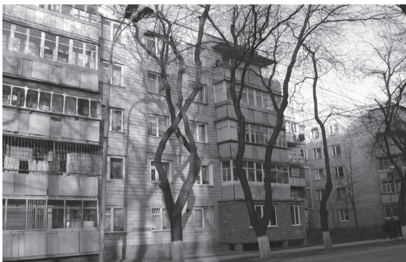
Fig. 6.9 Panel housing in Chisinau – home to owners and tenants
