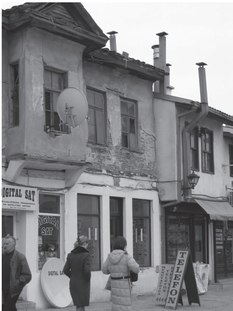
Fig. 10.6 Substandard housing in the historical district of Skopje
