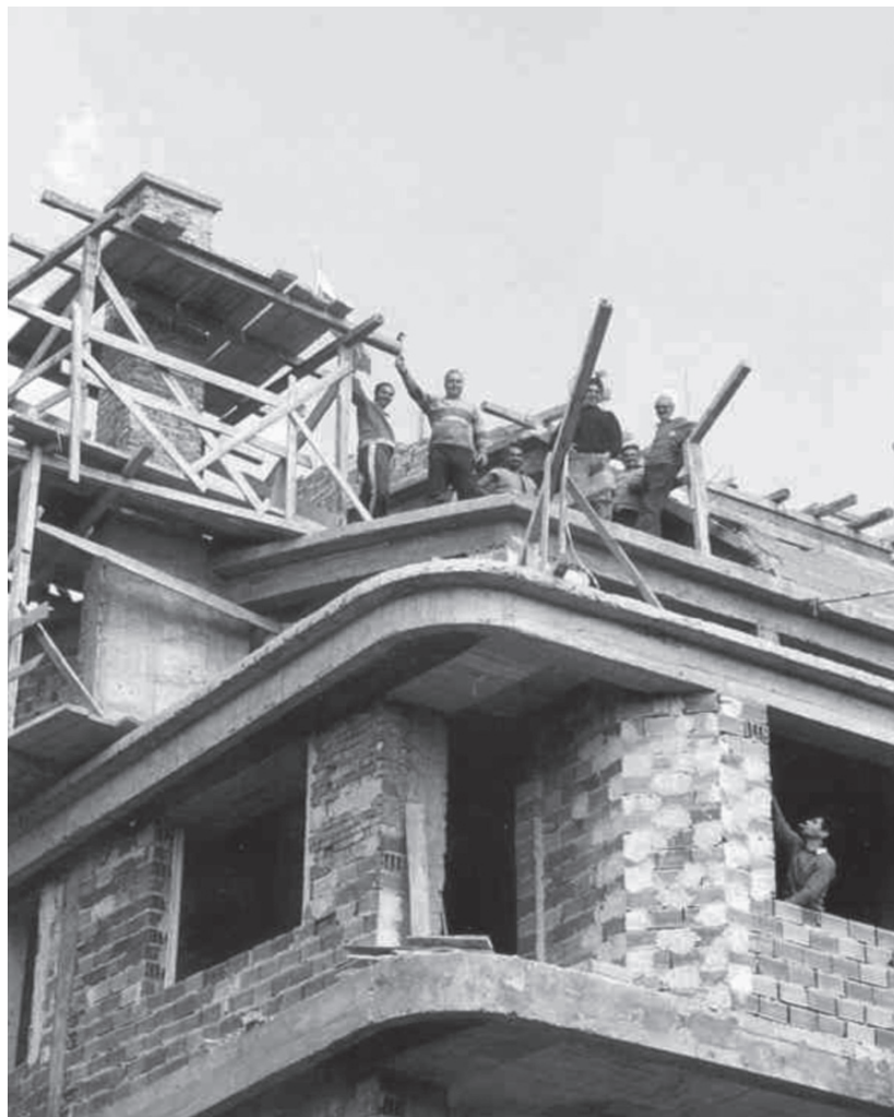
Fig. 1.3 New tradition built housing in Sofia, Bulgaria
