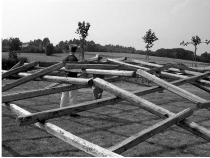
Fig. 4. First dome completed
