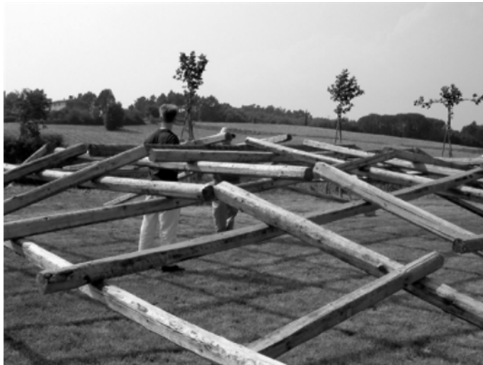
Fig. 4. First dome completed
