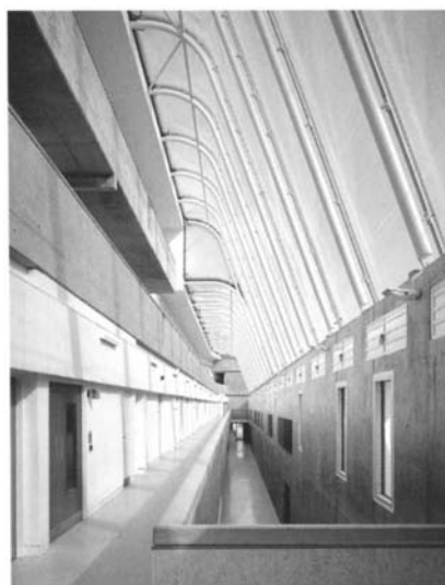
Internal views of ETFE atrium. Academy of St. Francis of Assisi, Liverpool
