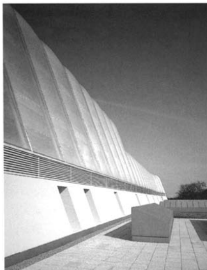
South-facing passive solar ETFE atrium. Academy of St. Francis of Assisi, Liverpool, Buro Happold
