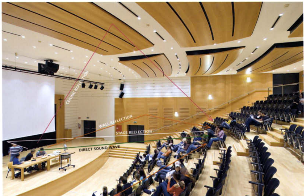
Details of elastic suspension of walls and ceiling in Aula Magna at Gasteiner Upper School Bolzano, South Tyrol, V. Andriolo, 2001
