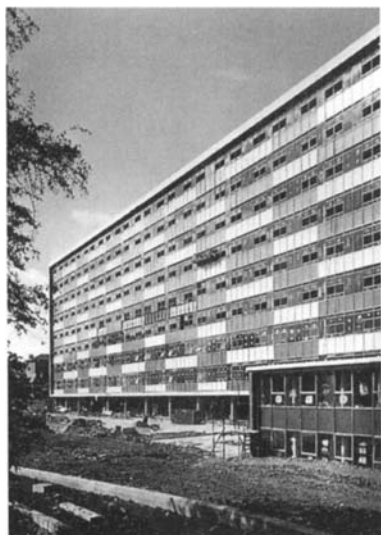
Tulsa Hill Comprehensive School London, London County Council, 1953-1966
