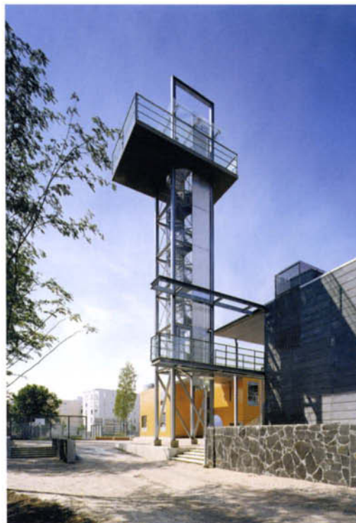
The lower school classrooms are in the yellow clad block | The observatory tower, a decorative feature which emphasises transparency | Main entrance orientated to the south with contrasting grey and brown cladding panels with the glazed atrium at the centre | Atrium with galleries | View inside the atrium looking down towards the main staircase
