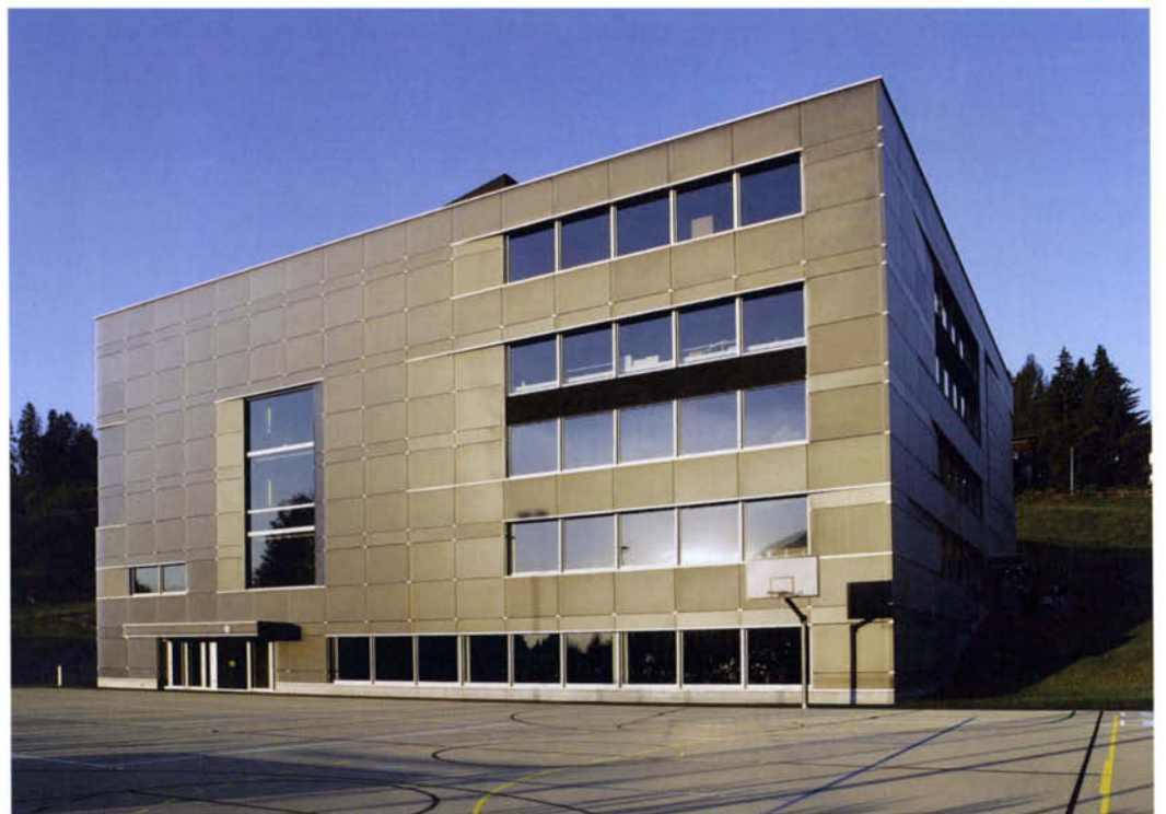
Site plan | Elevation to the south | Third floor view along corridor with bridge link connecting across to teaching spaces | View into gymnasium, the interface between the lower and upper schools
