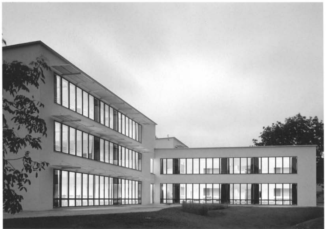
Typical south-facing windows showing alternate open and fixed glazed panels with projecting solar shading canopies | View of laboratory courtyard showing alternate three-storey wings and main block of accommodation
