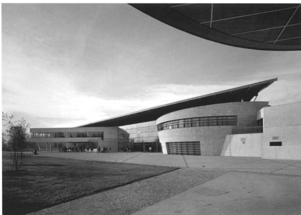
A bridge link across the courtyard gardens connects the teaching blocks | The main communal building with learning resources and social areas projecting out into the landscape | The entrance lobby with mezzanine bridge link | Typical internal corridor within the teaching blocks
