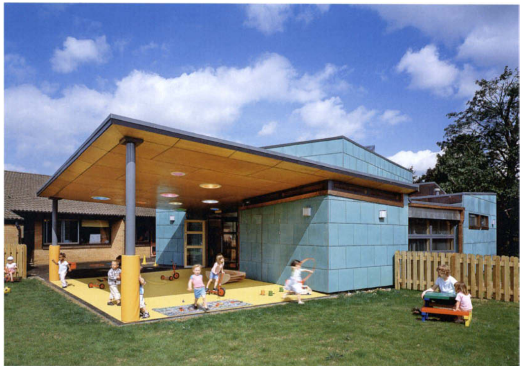
View of the main entrance showing the distinctive blockish form | View from the garden and outside play areas | Interior view of the main playroom area with the lower and higher ceiling planes giving spatial drama to the activity area | Coloured rooflights are only one of a number of child-orientated construction details which enhance the experience of play and learning
