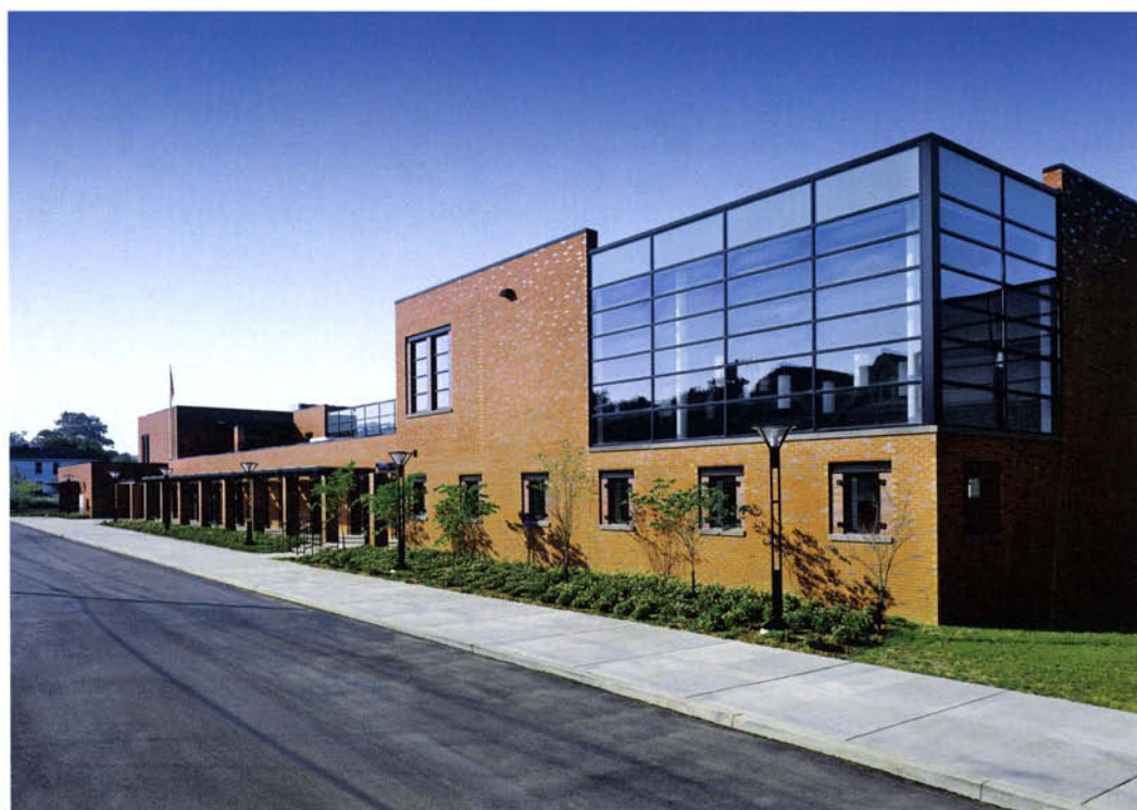
Internal courtyard showing external solar shading | Main entrance looking towards community café | Student and community ICT suite | Interior view of classroom break-out spaces
