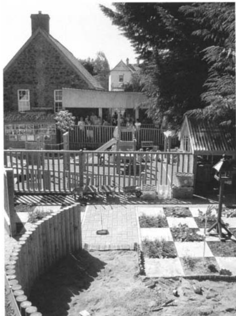
A limited budget spent on small-scale improvement raises the quality of the environment immeasurably. Nursery in Loup, Northern Ireland, 2005. Mark Dudek Associates, before and after refurbishment.
