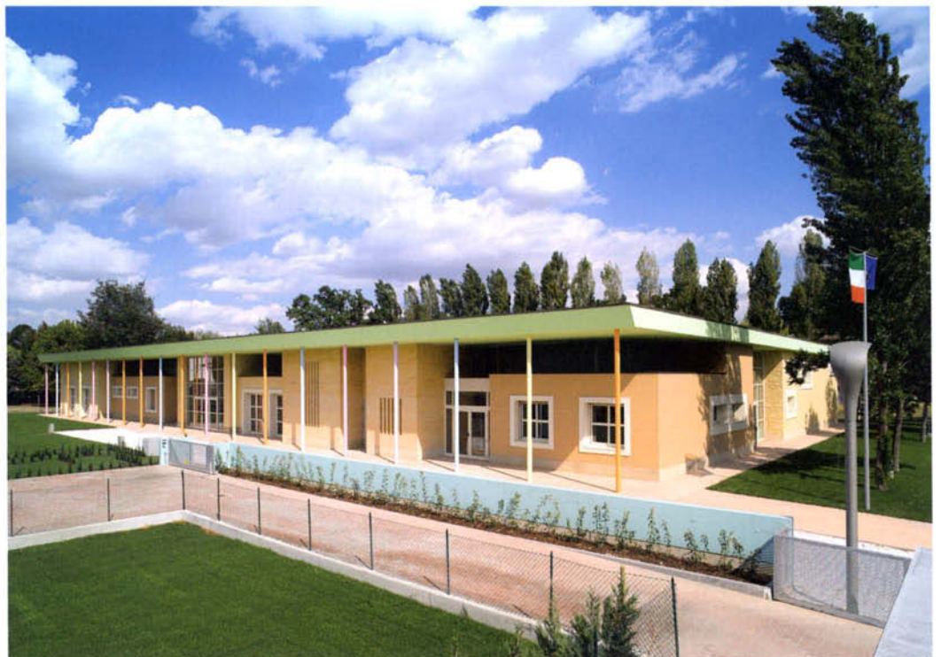
Views of covered colonnade providing a natural extension to the interior space out into the gardens | Night view | The central square with views to the courtyard garden, a little bit of outside space captured within the building
