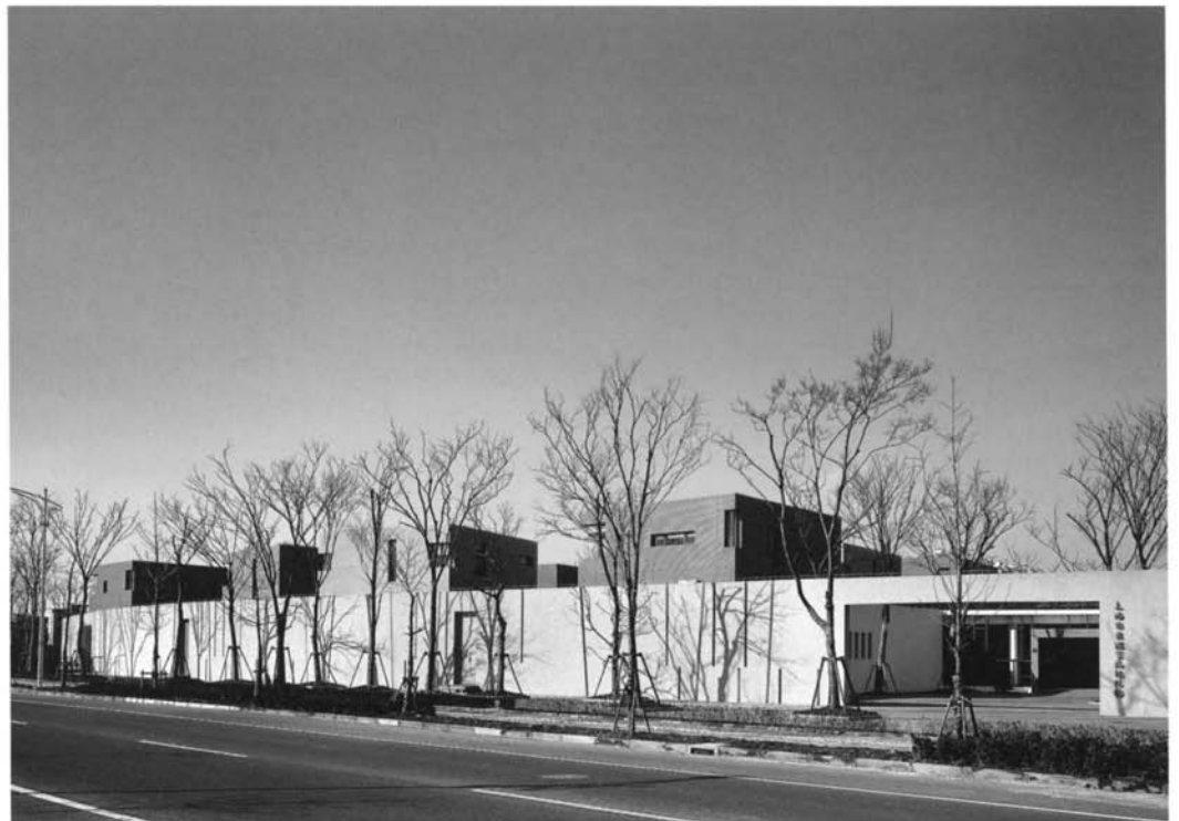
Glazed wall to office administration compound | The wall with children's houses peeking above | Roof walkway | View of corridor
