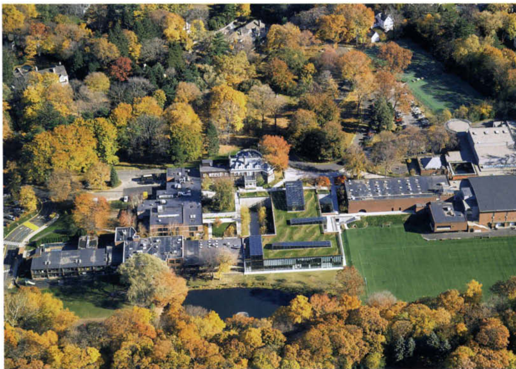
View of library courtyard, the axial view deliberately frames the historic buildings | Aerial view shows grass roof and the new building bridging between the existing buildings on site
