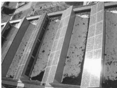
23.76 kW photovoltaic panels system. Academy of St. Francis of Assisi, Liverpool, Buro Happold
