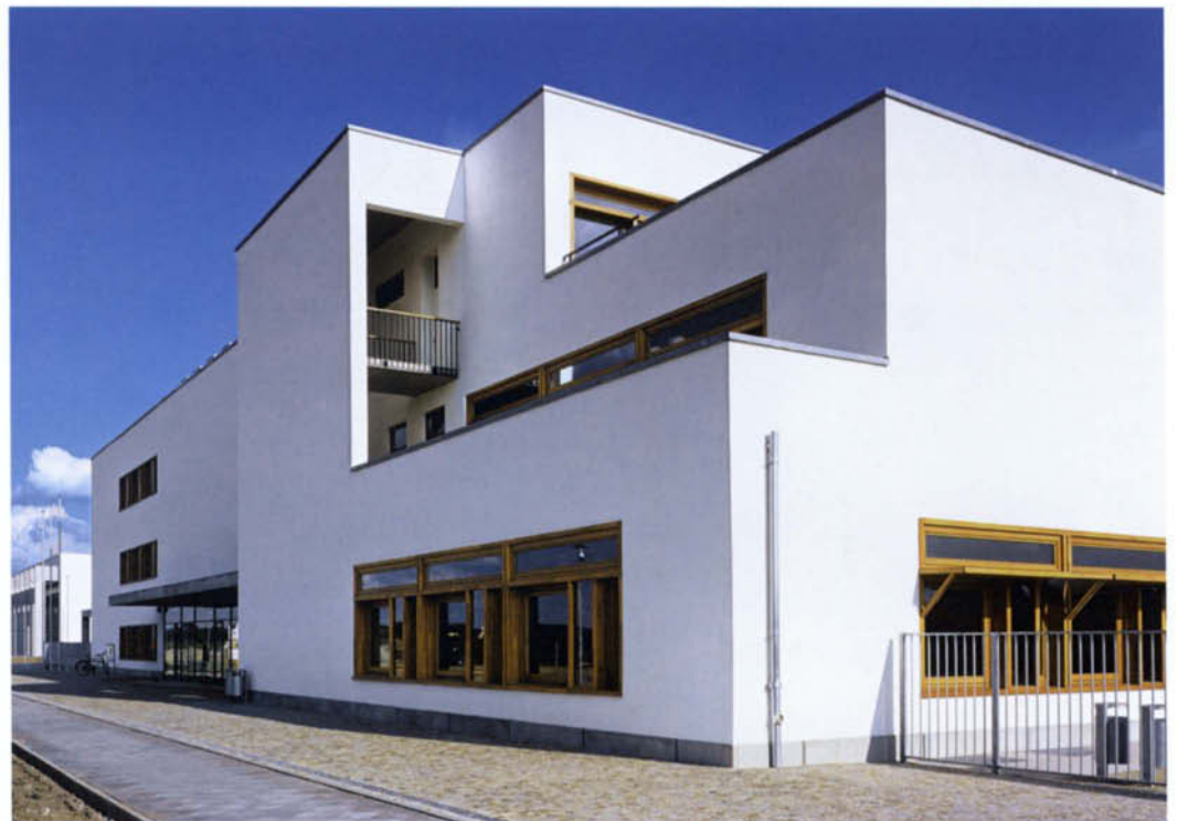
North-facing street façade | Courtyard with walkway to sports hall | Interior showing generous circulation area using natural materials and modulated lighting effects
