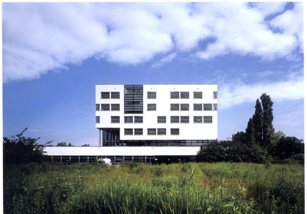
Entrance staircase | Lateral façade with technical classrooms in the 'base level' | View of central void | Grand staircase | Study area outside the classroom
