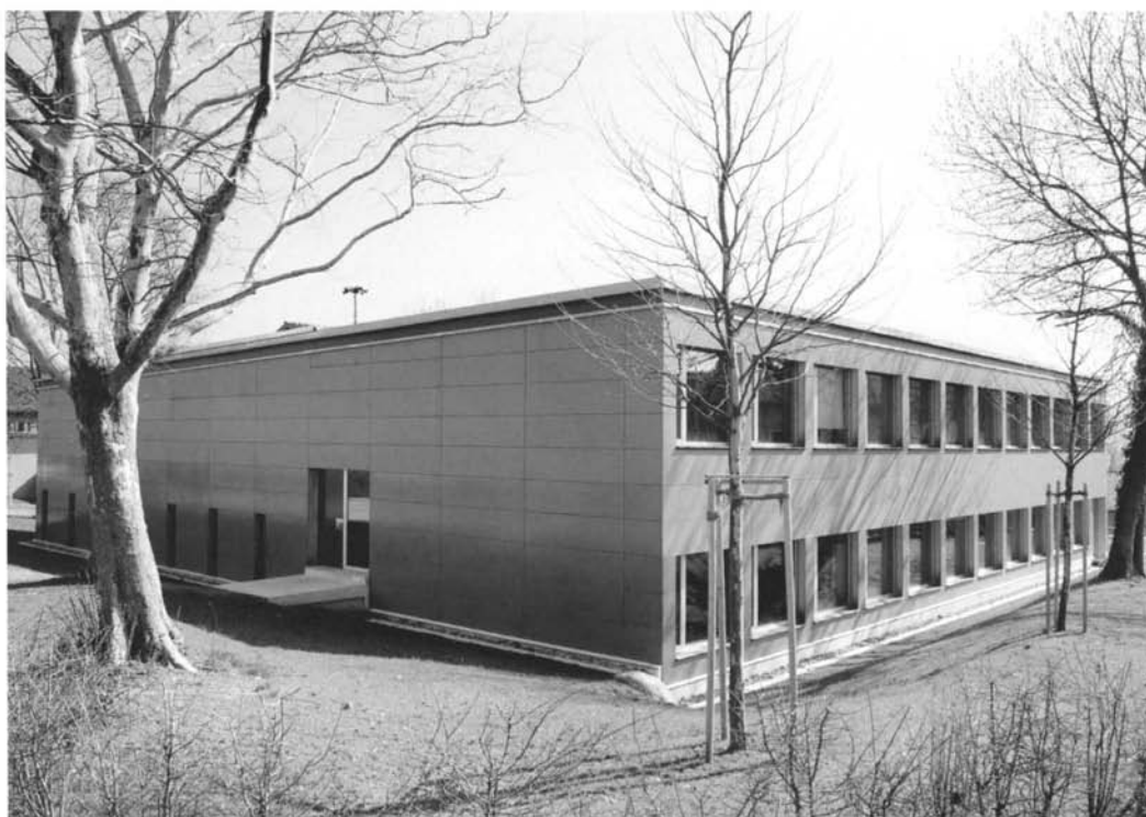
Terrace with new extension connected elegantly onto the existing building | View from northeast | Renovated classroom with coordinated furniture and timber wall paneling | Old building with new corridor façade with integrated storage and pupil lockers
