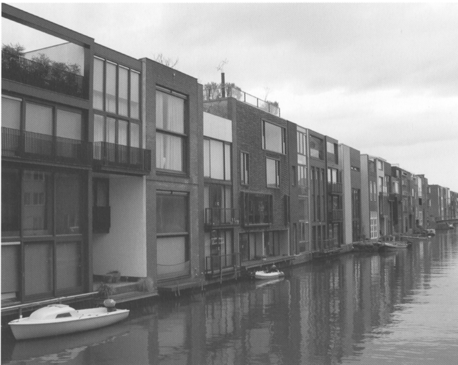
Several row houses, Amsterdam
