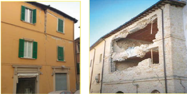
Figure 4. Out of plane rocking.
