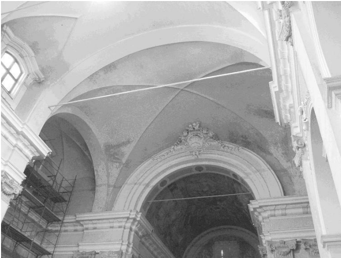
Figure 5. The roof vault of the presbytery area.
