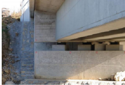
Fig. 7 Elastomeric support inserts under the deck
