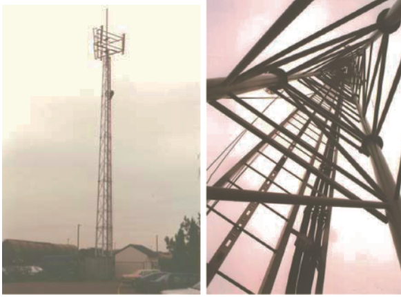
Figure 14. Steel mast with sectorial antennae at the top.
