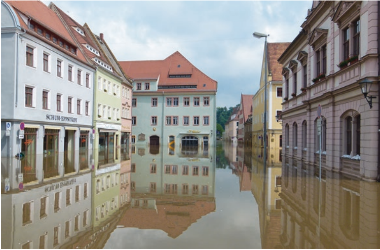
Fig. 6.5 Elbe flood 2002 in Pirna. (Photo © Haase)
