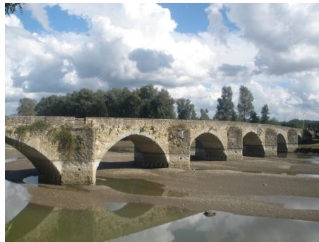
Fig. 2. The bridge crossing Arno in Arezzo
