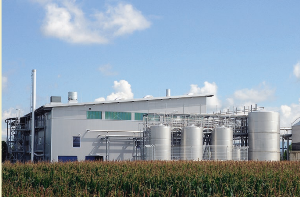
Demonstration plant for the production of 2G-ethanol based on straw in Straubing, Bavaria. The Clariant Produkte Deutschland GmbH plant has a production capacity of 1000 t ethanol per year. (© Clariant)
