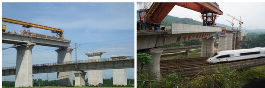
Fig. 9.2 Construction of a new bridge crossing the existing railway (City8 2015)
