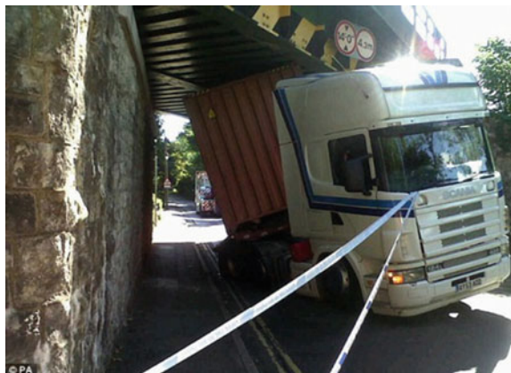
Fig. 1.24 Railway bridge hit by truck in England (dailymail 2011)
