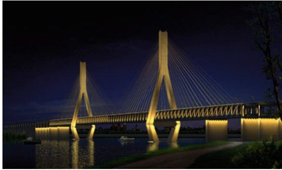
Fig. 1.8 Wuhan Tianxinzhou Yangzi River Bridge (blog. alighting 2012)
