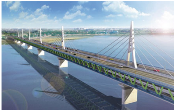
Fig. 1.9 Zhengzhou Yellow River Rail-cum-Road Bridge (Zheng et al. 2008)
