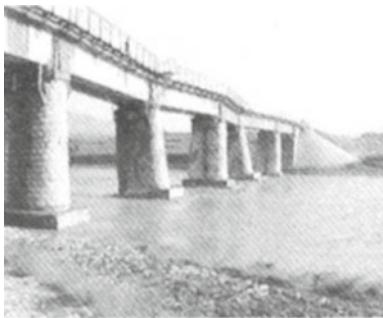
(a) the Dongquan River Bridge
