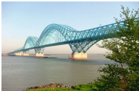
Fig. 1.7 Nanjing Dashengguan Yangzi River Bridge
