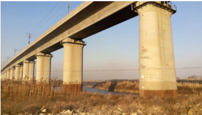
Fig. 9.45 Second Songhua River Bridge on Harbin-Dalian HSR
