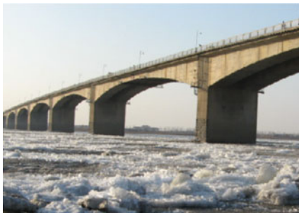
Fig. 8.20 Ice-floes drifting on the Tonghe Songhua River and a 90 m × 90 m floe colliding with the No. 38 pier of the bridge (maximum impact force 315.83 kN)
