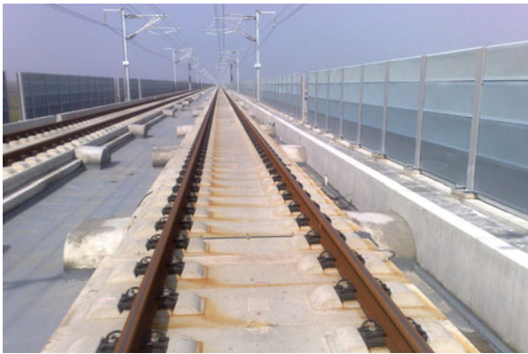
Fig. 10.37 CRTSII ballastless slab track on the bridge
