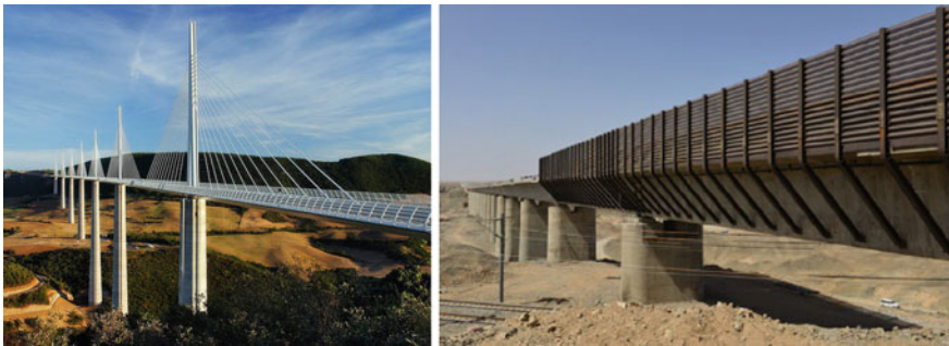
Fig. 6.1 Grille wind barriers on the Millau Viaduct in France ( left , highestbridges 2004) and plate wind barriers on a bridge of the Lan-Xin HSR ( right )
