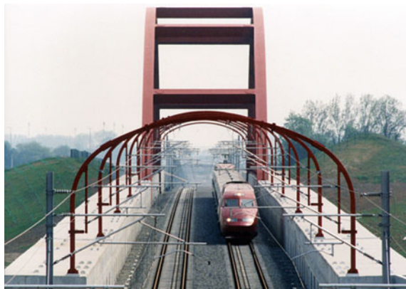
Fig. 1.29 Thalys train running through a HSR bridge (Belgium)
