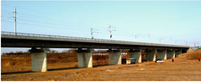
Fig. 5.14 View of the Gouhe Bridge on the Qin-Shen HSR line
