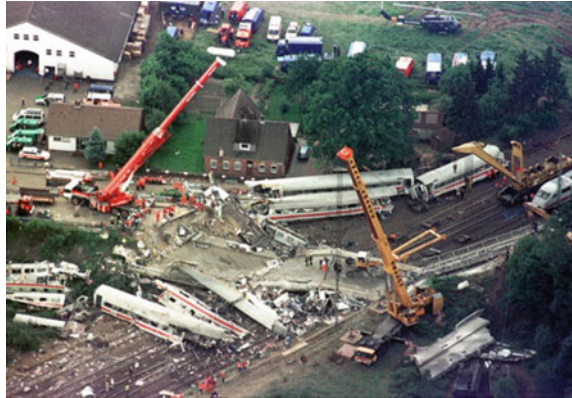
Fig. 1.23 Derailed ICE train and collapsed bridge (blog. sina 2011)
