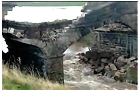
(b) the brick-arch bridge on Feltham Railway (England)
