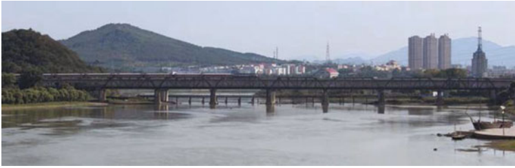
Fig. 9.47 The river-crossing section of the Mudanjiang River Bridge
