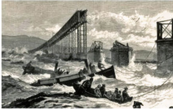
Fig. 1.12 Wind-induced accident of Tay Rail Bridge in Scotland (wikipedia 2016)
