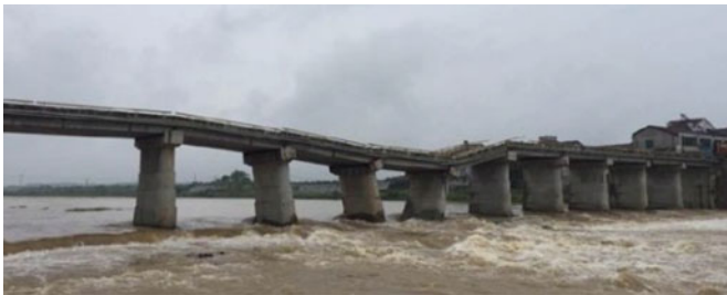
(c) the Huangkou Bridge on Yougang River
