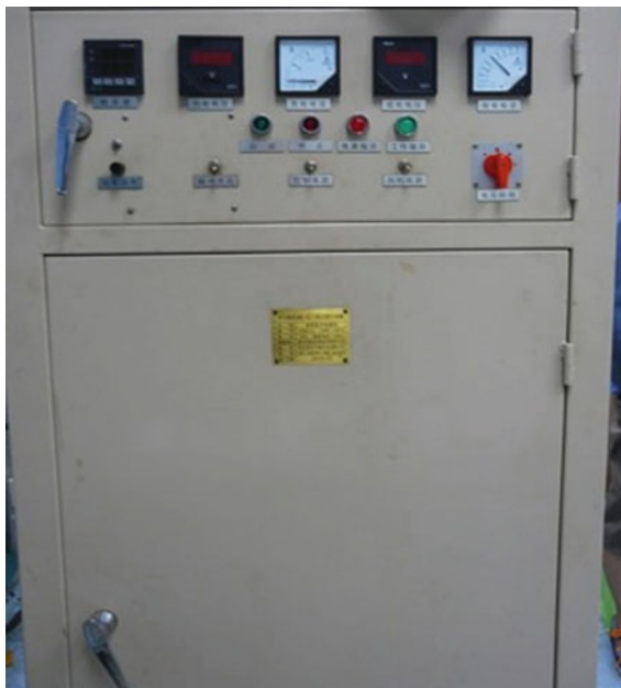
Fig. 6.1 AC electropulsing generator
