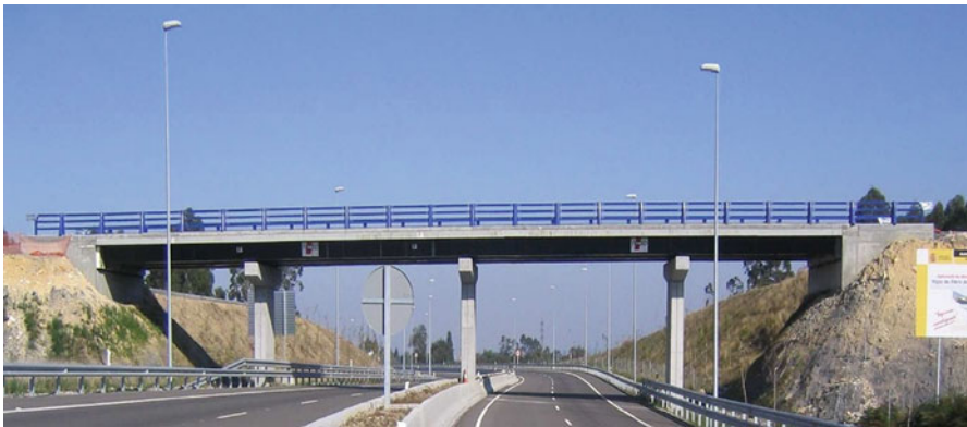
Fig. 3.12 Carbon fiber bridge in Spain [14Bus]
