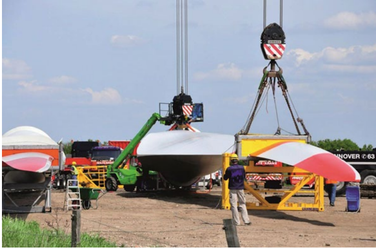
■ Fig. 9.3 The prototype of the rotor blade is prepared for installation. © Senvion GmbH 2015
