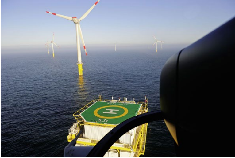
■ Fig. 1.4 Helicopter in landing approach to the helideck of the substation at the Alpha Ventus offshore wind farm. © DOTI/Alpha Ventus (Photographer: Mathias Ibeler)
