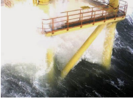
▣ Fig. 3.7 A 12-metre-high wave hits the Fino 1 research platform. Extreme sea state events have an impact on the logistics and plant management of offshore wind farms. © DNV GL
