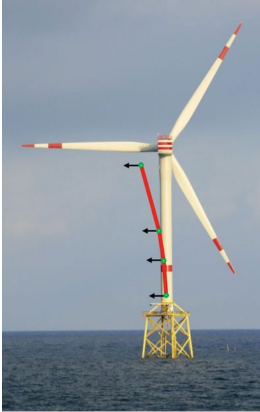
■ Fig. 5.2 Monitoring the condition of the turbine with modal parameters from the long-term measurements. © Senvion GmbH 2015
