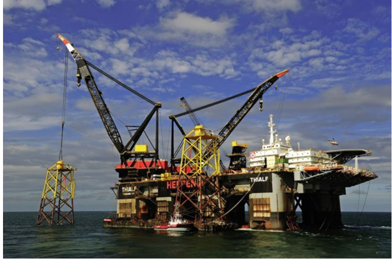
Fig. 1.3 The pontoon crane Thialf installs a jacket foundation in the Alpha Ventus construction site. © DOTI/ Alpha Ventus (Photographer: Mathias Ibeler)
