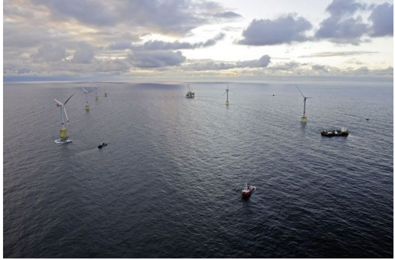
Fig. 1.1 A bird's eye view of Alpha Ventus during construction. © DOTI/Alpha Ventus (Photographer: Mathias Ibeler)
