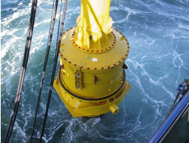
■ Fig. 22.5 The “bubble curtain” method of reducing noise surrounds the pile with fine air bubbles while the hydraulic piledriver hammers the pile into the seabed. © LUH
