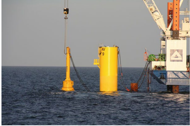
■ Fig. 22.1 The Menck MHU 800S hydraulic ram used at the Alpha Ventus offshore wind farm. © Menck GmbH
