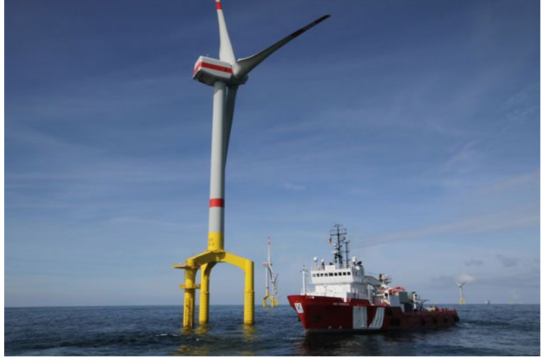
■ Fig. 7.1 Offshore wind turbines with tripile foundations. © Ocean Breeze Energy GmbH & Co. KG
