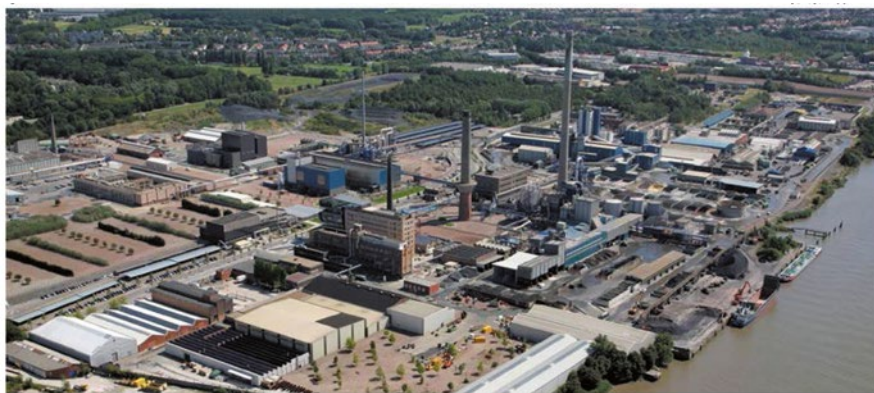
Fig. 27.1 Umicore in Hoboken, Belgium. The largest recycling plant of its kind worldwide, it handles more than 350,000 t per year of source material [1]
