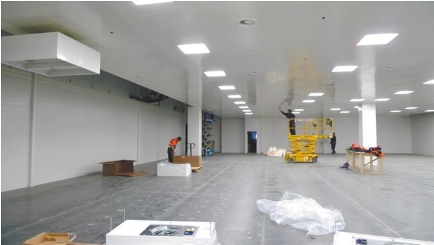
Fig. 18.4 Dry room for mass production under construction (Source M+W Group)
