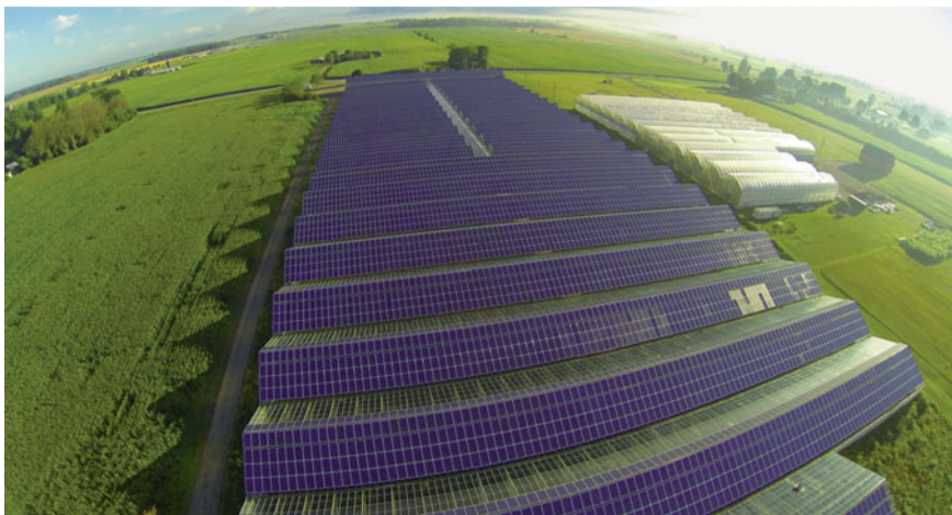
Fig. 5 A photo of 2.3 MW micro-inverter solar project at Ontario, Canada’s Vine Fresh Produce
