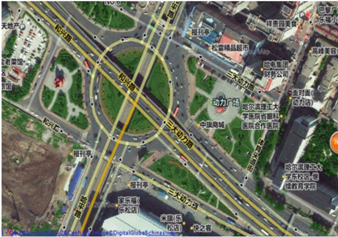
Fig. 53.1 Roundabout of Dongli square in Harbin
