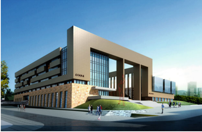
Fig. 22 A school building in Guizhou University
