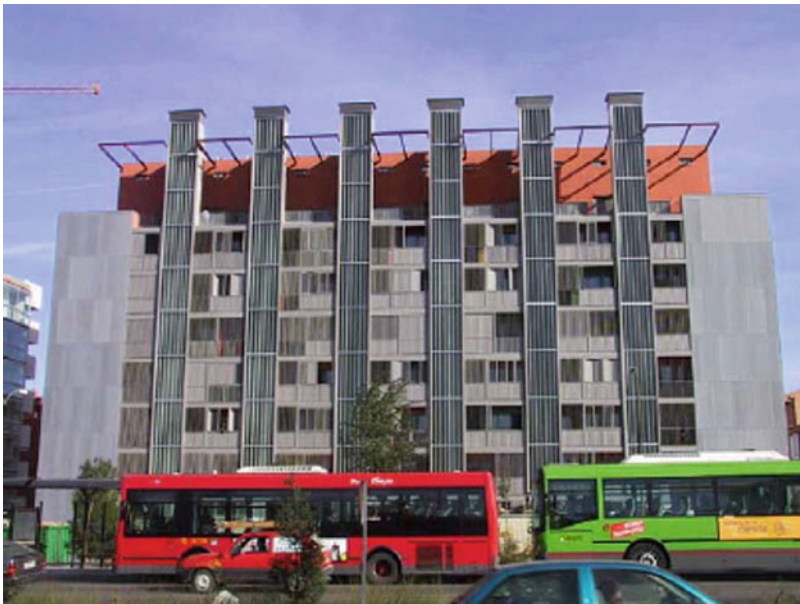
Fig. 10 West facade with solar chimneys of the building [24]
