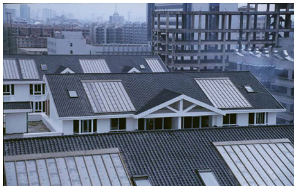
Fig. 35 Solar collectors were imbedded into roofs of buildings in Kunming (Courtesy of Xinyuan Sunlight Co)
