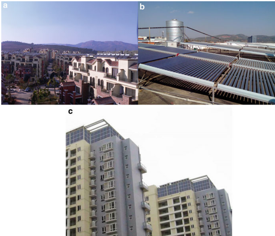
Fig. 21 (a) Domestic solar water heaters, (b) collective solar hot water supply system, (c) collective-individual hot water supply system
