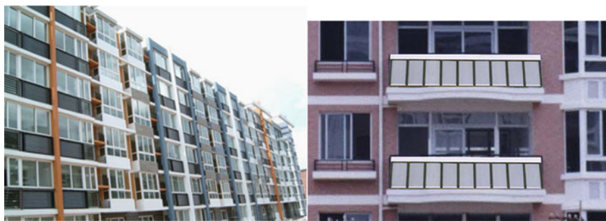
Fig. 36 Solar collectors integrated into balcony and walls of buildings (Courtesy of Xinyuna Sunlight Co)
