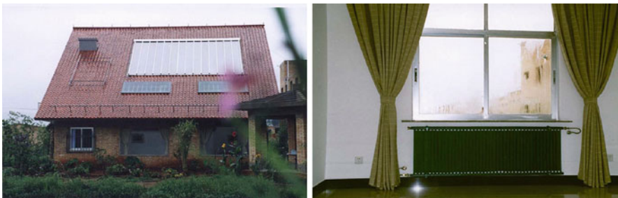
Fig. 34 Left: South-roof partially covered by solar collectors. Right: Bedrooms heated by the solar water heating system (Courtesy of Xinyuan Sunlight Co)
