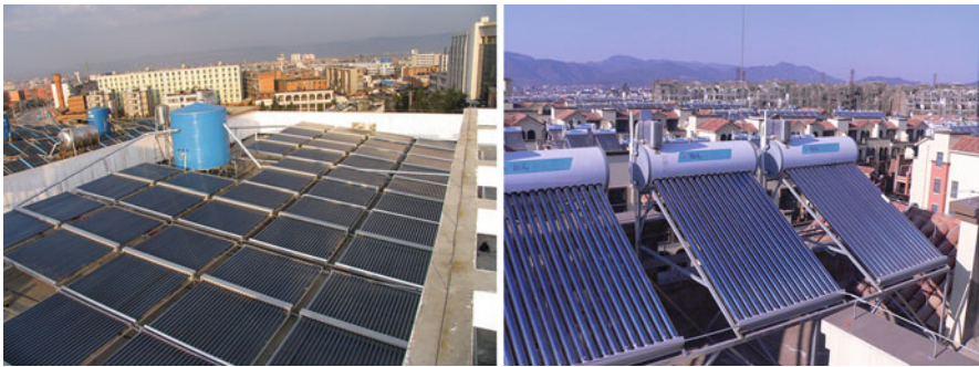
Fig. 11 Left: H-type collector; right: T-type collector (Courtesy of Xinyuan Sunlight Co., Yunnan of China)
