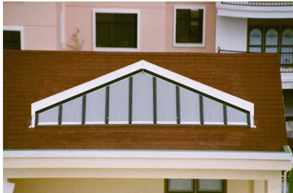
Fig. 38 Solar collectors as the sky-light of living rooms (Courtesy of Xinyuan Sunlight)
