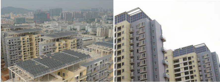
Fig. 40 Collective hot water supply systems. Left : collectors on roof, right : part of collectors on southern wall
