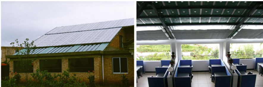
Fig. 33 Left: South-roof covered by solar water modules; right: holes on the solar collector modules provide daylight to the office (Courtesy of Xinyuan Sunlight Co)
