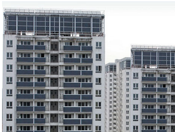
Fig. 40 Collective hot water supply systems. Left : collectors on roof, right : part of collectors on southern wall
