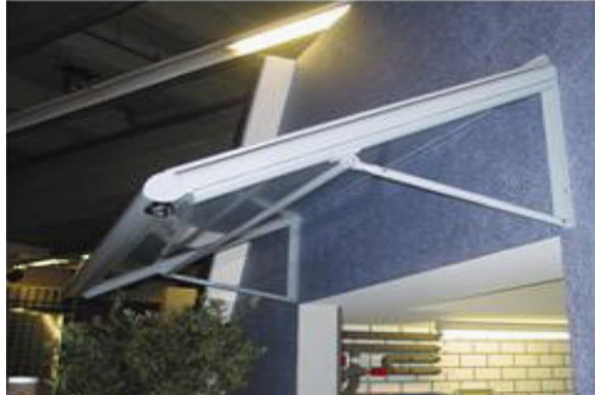
Fig. 37 Solar collectors as the overhang shelter of windows
