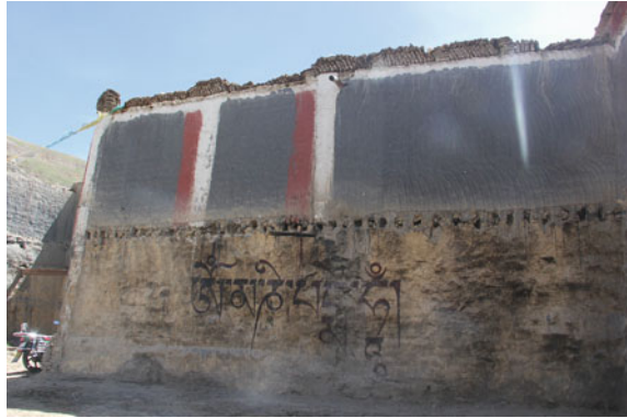
Fig. 9.4 Decorative patterns of residential buildings (Source ©Authors)
