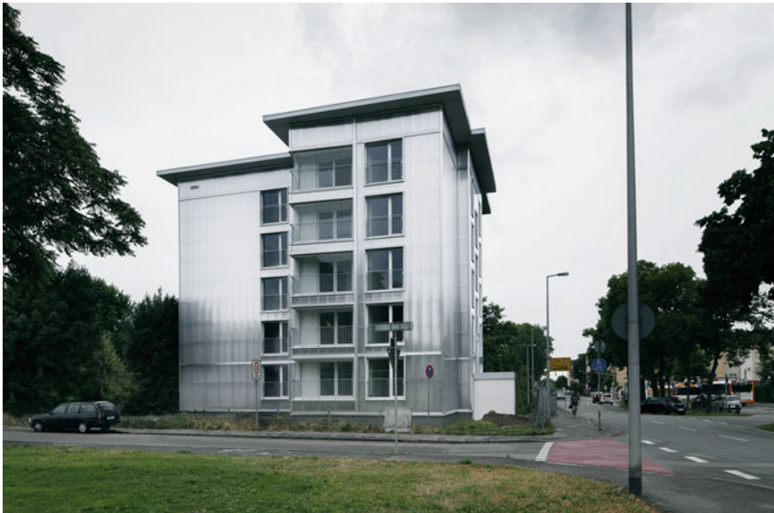
Fig. 4.8 Social housing after renovation in 2014, ©Claudius Pfeifer
