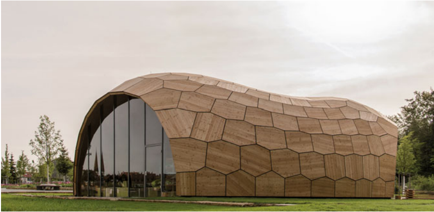
Fig. 7.8 The Landesgartenschau Exhibition Hall is a demonstrator building for the research project “Robotics in Timber Construction” (Source ICD/ITKE/IIGS University of Stuttgart)
