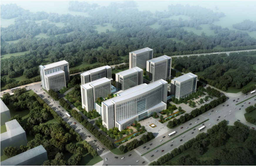
Fig. 8.12 Haihu New District Hospital (2000 beds), Xining City, Qinghai (Source IPPR)
