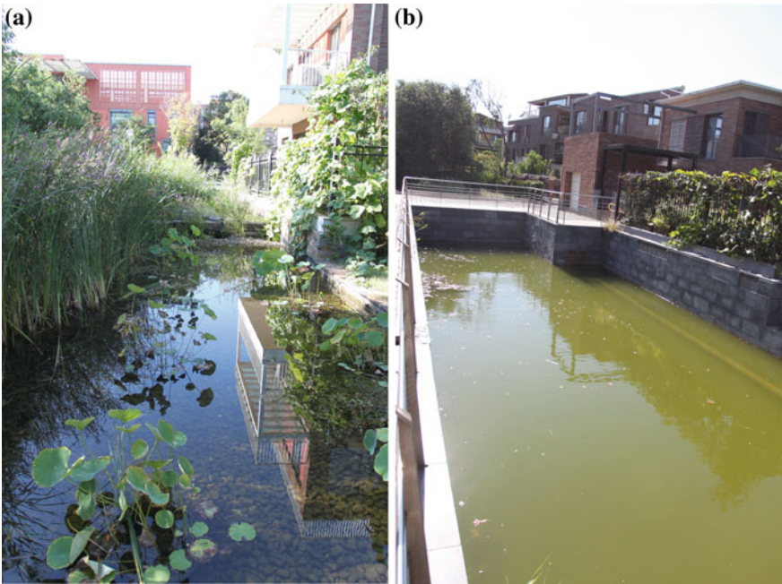
Fig. 1.16 a, b Transforming existing canals and ponds for the contemporary stormwater management (Source Li Xin)
