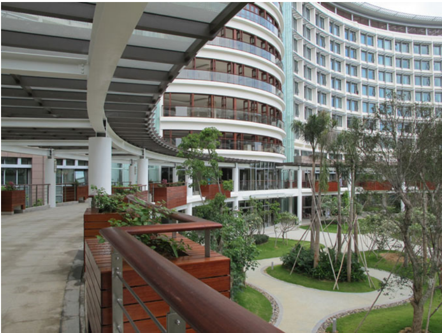
Fig. 8.29 Exterior courtyard (Source IPPR)
