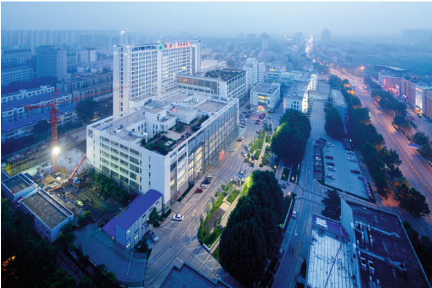
Fig. 8.2 Hebei People's Hospital, Shijiazhuang City, Hebei (Source IPPR)
