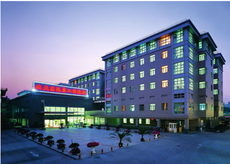
Fig. 8.6 Peking University First Hospital, Beijing ( Source IPPR)
