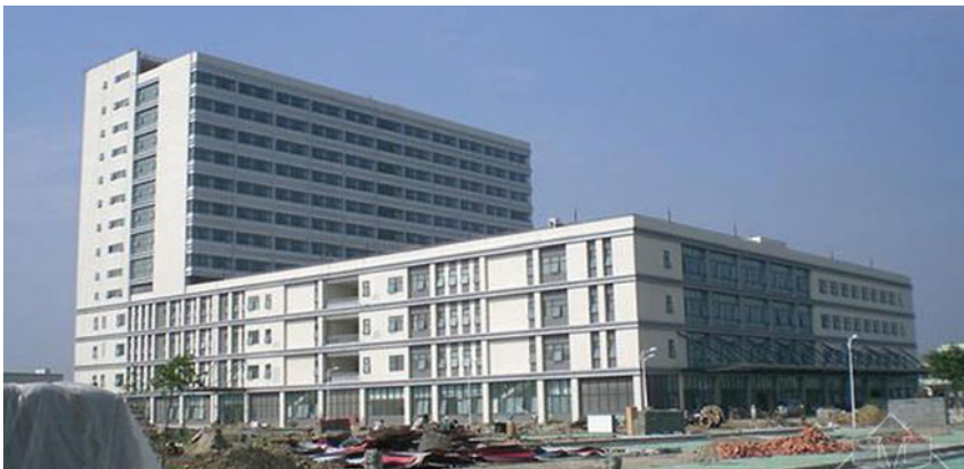
Fig. 8.15 Peoples’ Hospital, Shifang City, Sichuan (Photo taken on-site, Source IPPR)
