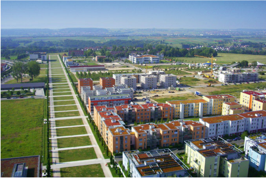
Fig. 1.2 Scharnhauser Park during construction, showing the orientation of the landscape staircase towards the surrounding hills ( Source SEG Ostfildern)
