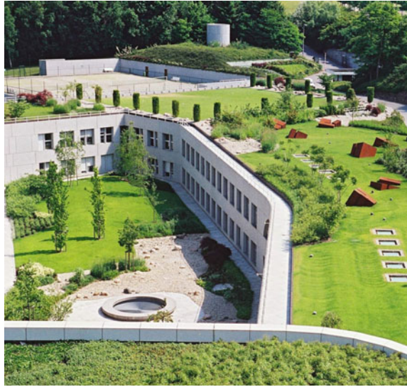
Fig. 17.6 Green roof in Beijing. Source http://www.cqla.cn/chinese/news/news_view.asp?id=26414
