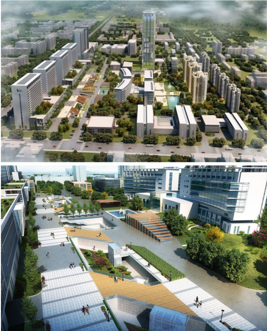
Fig. 8.21 Honliv Medical City, Xinxiang City (Source IPPR). *The project not only stimulates the development of residential, commercial, and senior living industries but also helps raise the living quality of local residents
